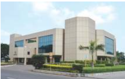
SBU Block (2nd floor), Hazira
