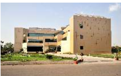
Administrative Building, LTSSHF, Hazira
