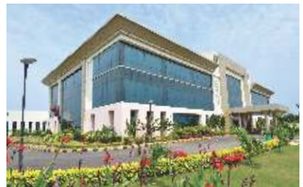
Administrative Building, Vadodara
