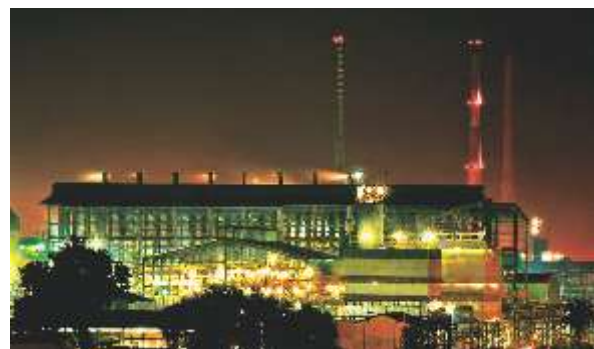
Complete Industrial Electrification solutions by L&T at Hindustan Zinc Ltd., Chanderiya, Rajasthan
