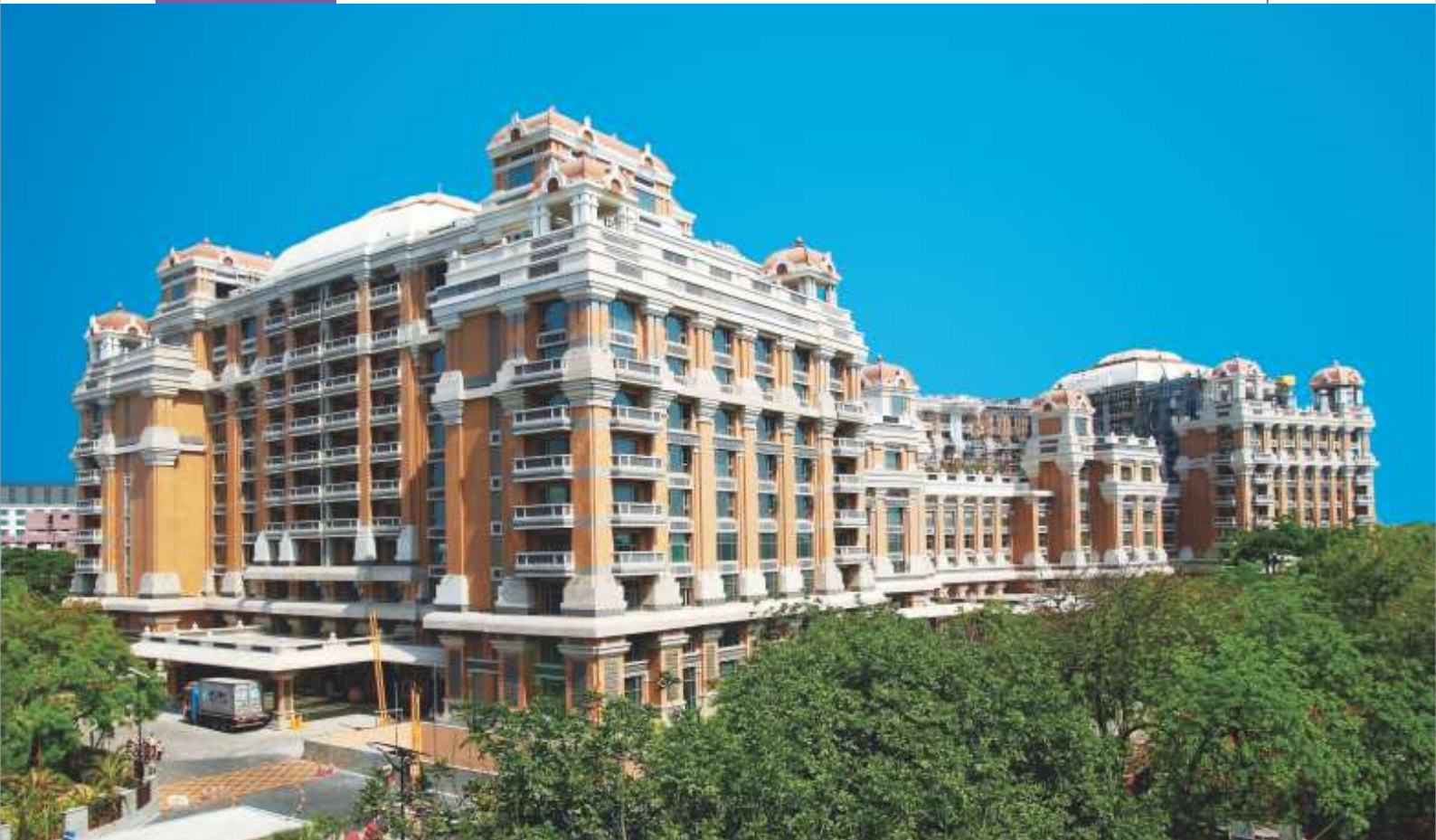
L&T has constructed ITC's 600-room five-star hotel – the world's largest LEED-certified green hotel
