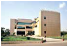
Administrative Building, LTSSHF, Hazira
