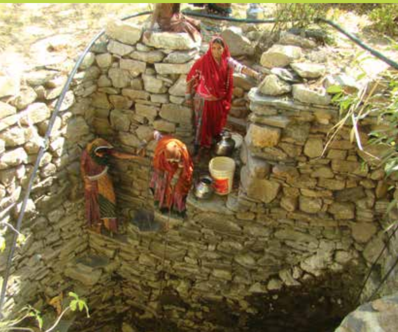
Before: Haraj village before L&T's intervention
