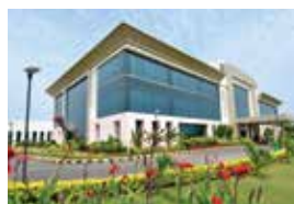
Administrative Building, Vadodara
