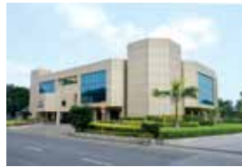
SBU Block (2nd floor), Hazira
