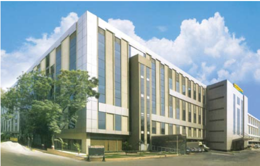
Powai Switchgear Factory, Mumbai.
