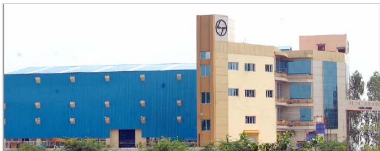
A view of the Service Centre.
