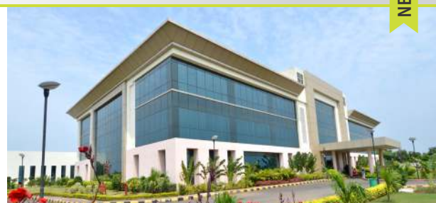
Administrative Building, Vadodara
