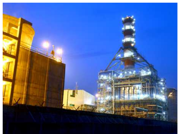
Power Plant at Dhuvaran, Gujarat
