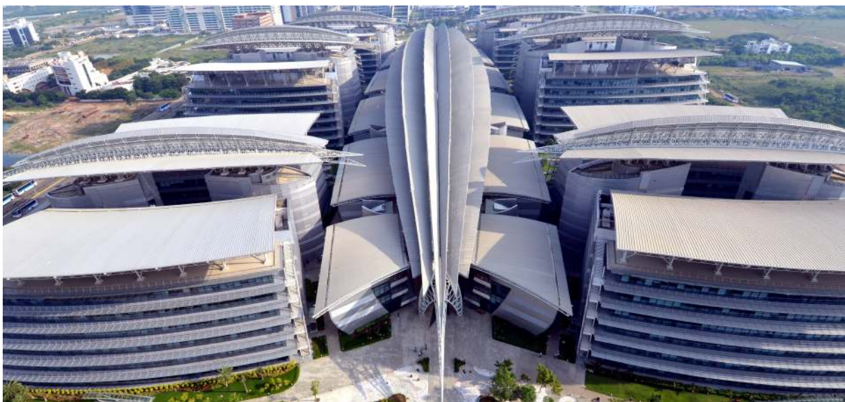
TCS, Seruseri Campus constructed by L&T
