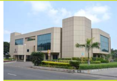
SBU Block (2 nd floor), Hazira
