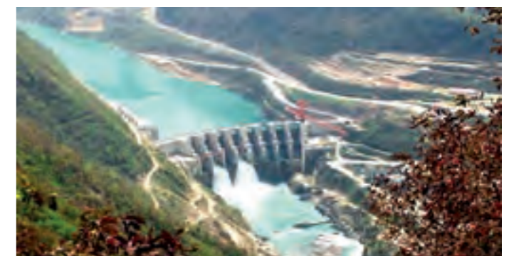
330 MW hydro-electric project in Uttarakhand - one of the many at the foothills of the Himalayas.
