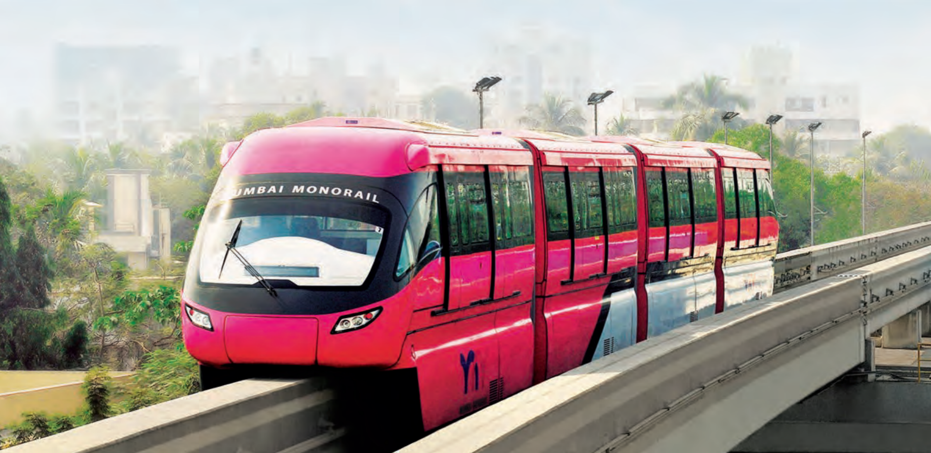
India's first monorail, at Mumbai, built and commissioned by L&T.
