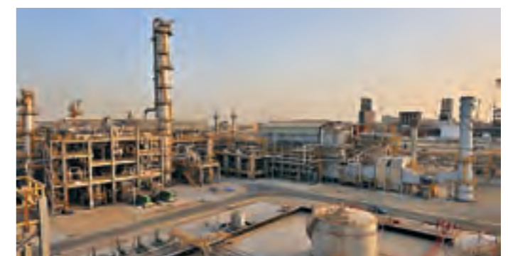
700 TPD Methanol + 100 TPD CO plant for Methanol Chemicals Company (CHEMANOL) at Al Jubail in Saudi Arabia.
