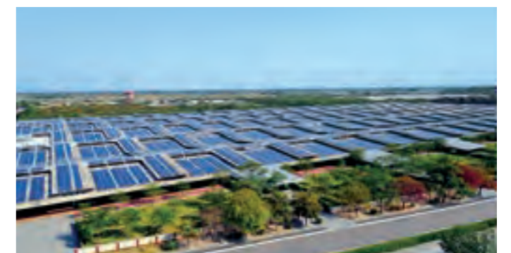
7.5 MW Solar PV plant on a single roof - one of the world's largest projects of its kind.
