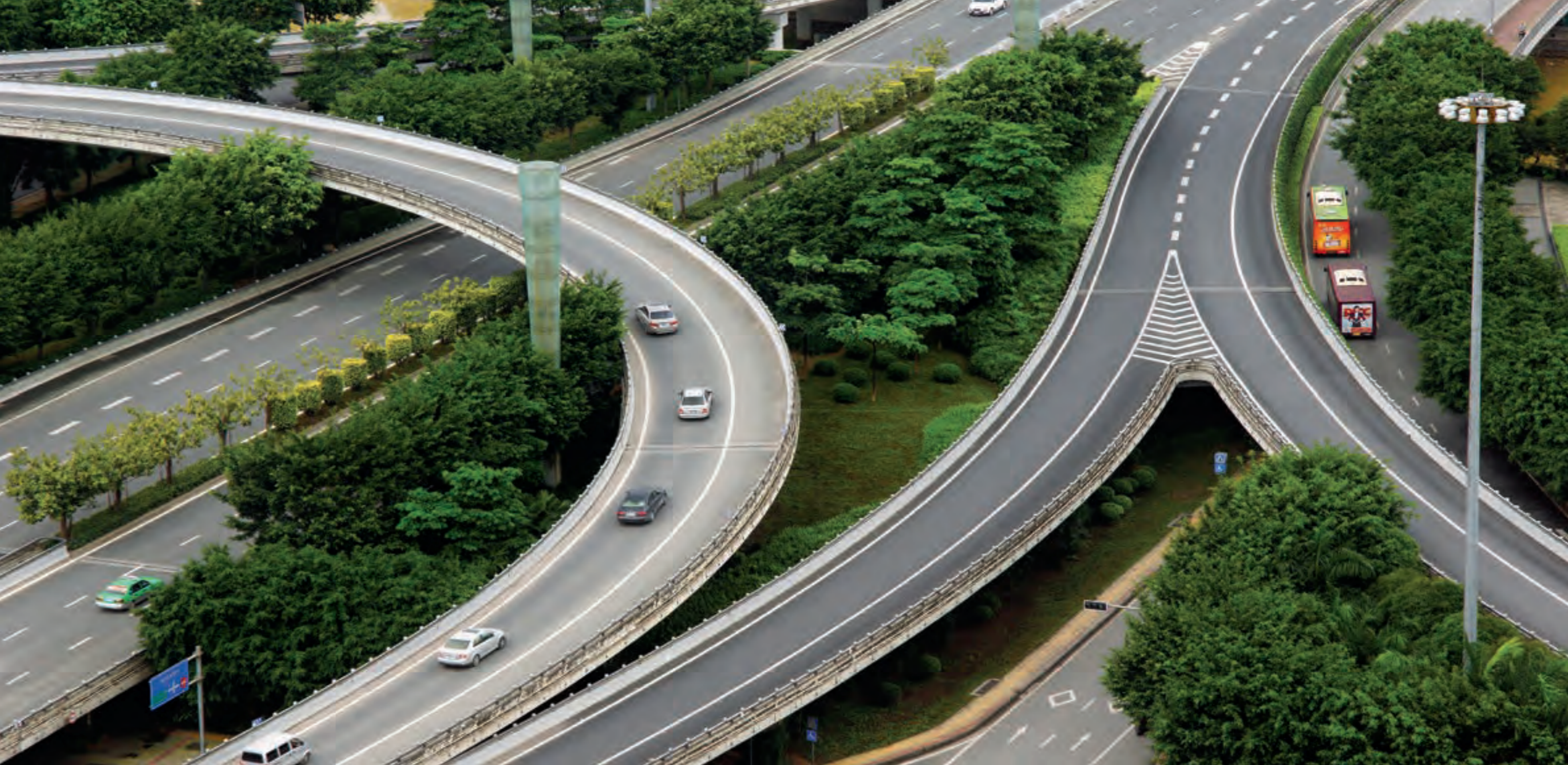
L&T is undertaking complex roads and interchange projects in several geographies. The track record includes the prestigious Sheikh Khalifa Interchange linking the emirates of Abu Dhabi and Dubai.
