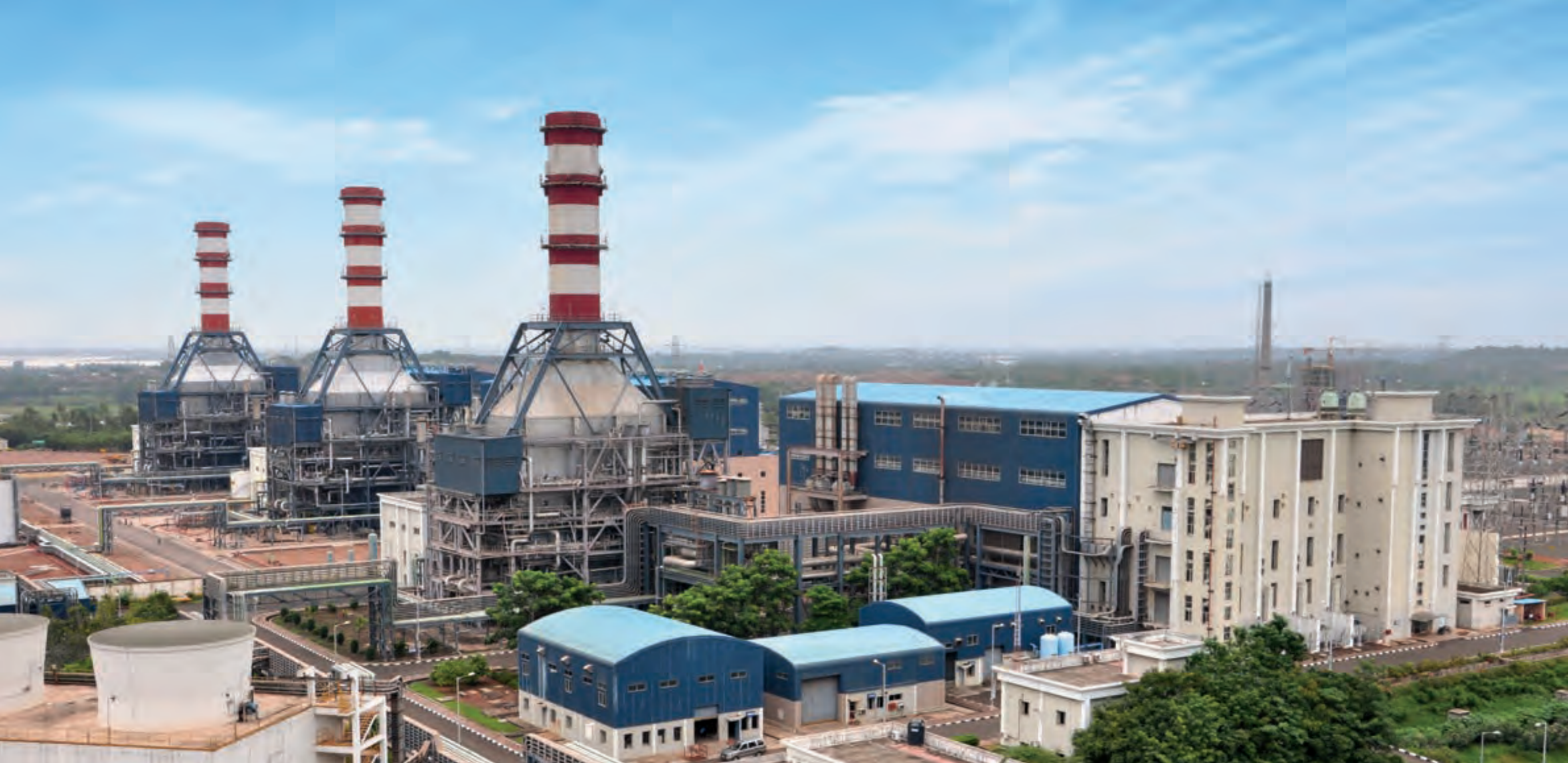
Natural gas-fired combined-cycle power plant built by L&T at Vemagiri in Andhra Pradesh.
