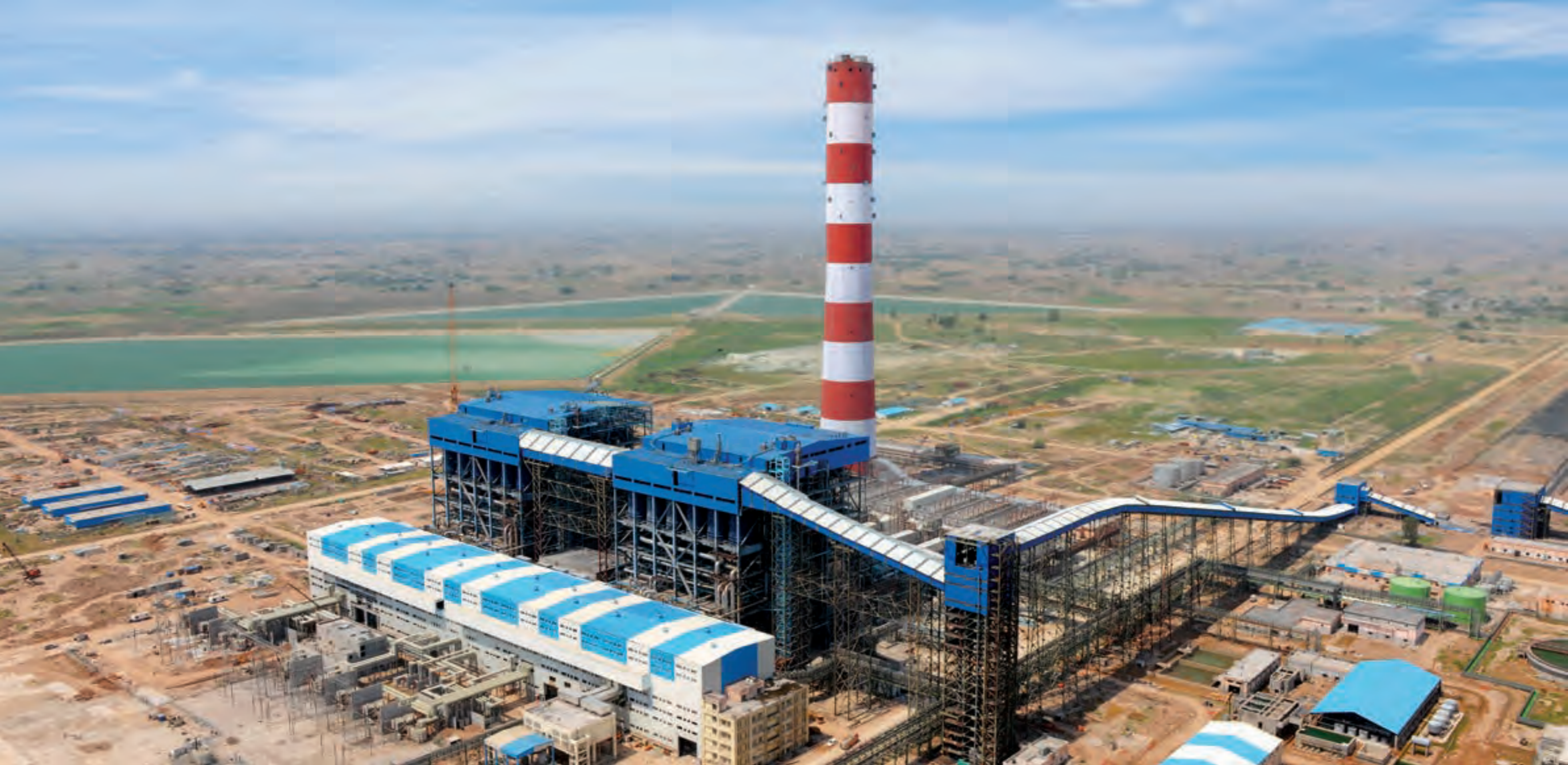
2x700 MW supercritical thermal power plant built by L&T on EPC basis for Nabha Power at Rajpura in Punjab. L&T's joint venture with Mitsubishi Hitachi Power Systems enables the power sector to access the advantages of world-class technology.
