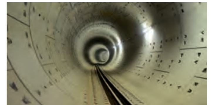
Tunnel for a major metro. L&T has also built underground and elevated corridors for the metro in major cities.
