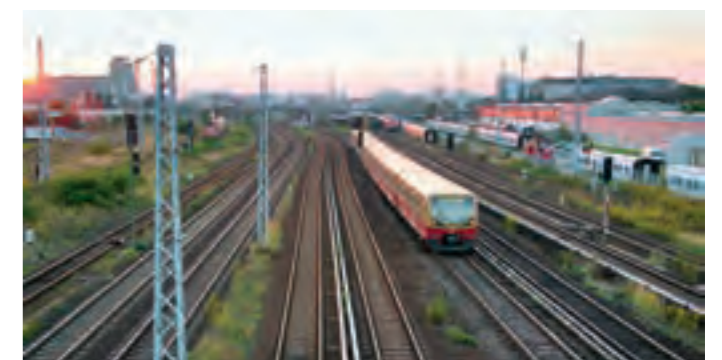
L&T is executing multiple integrated rail infrastructure projects, including the Dedicated Freight Corridor in India.
