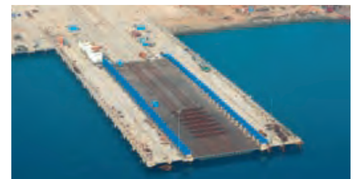
L&T's shipyard at Kattupalli on India's east coast, equipped with a shiplift designed and built in-house.
