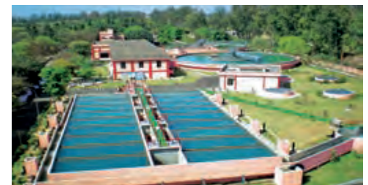
16 MGD water treatment plant for Delhi Jal Board. Since 2001, L&T has executed 13 water projects in India's capital.
