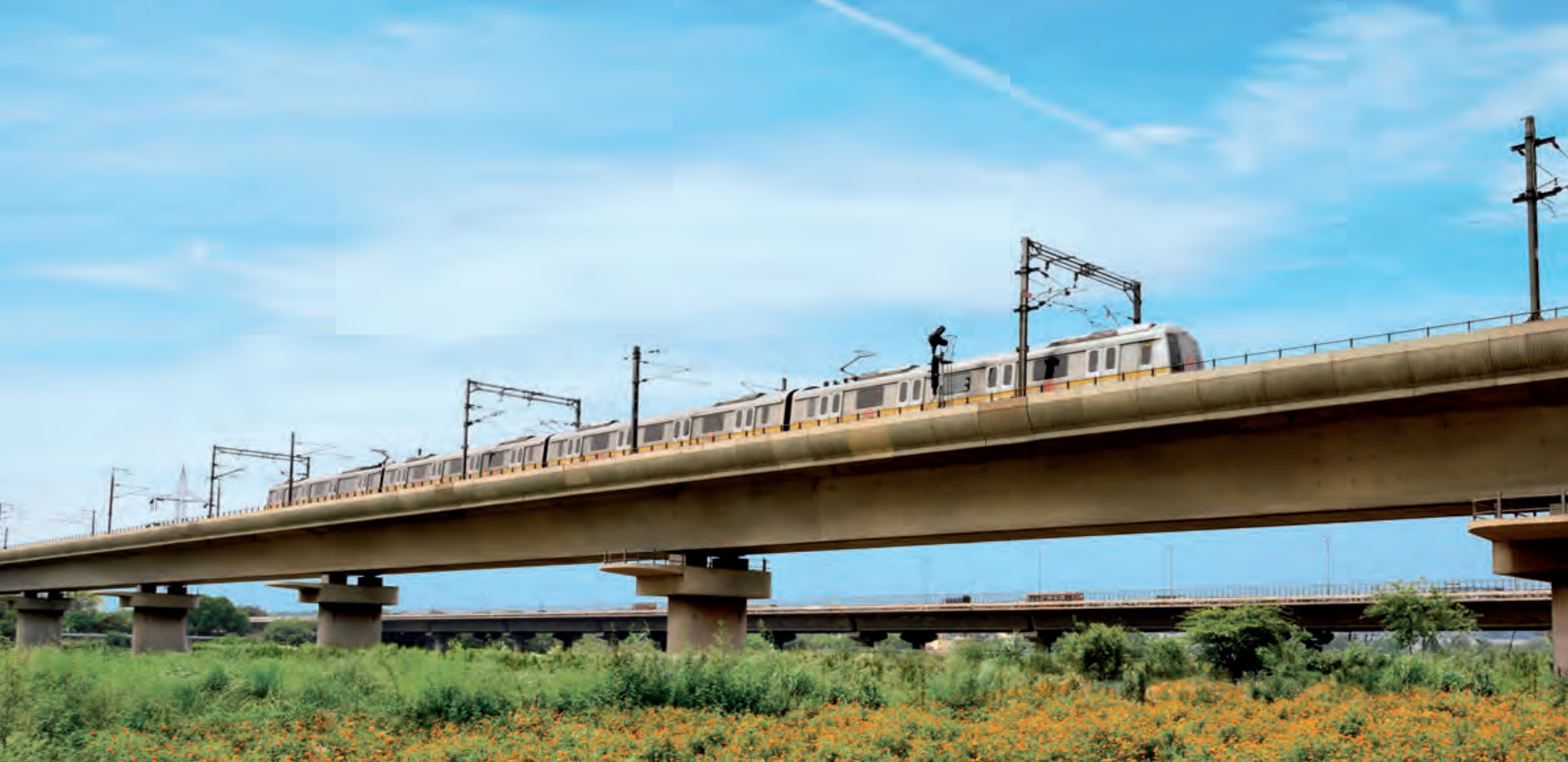
L&T has executed elevated and underground corridors and many station buildings with electrical & automation systems for Delhi Metro. L&T's metro profile extends across Riyadh, Qatar, Hyderabad, Kochi, Chennai and Bangalore.
