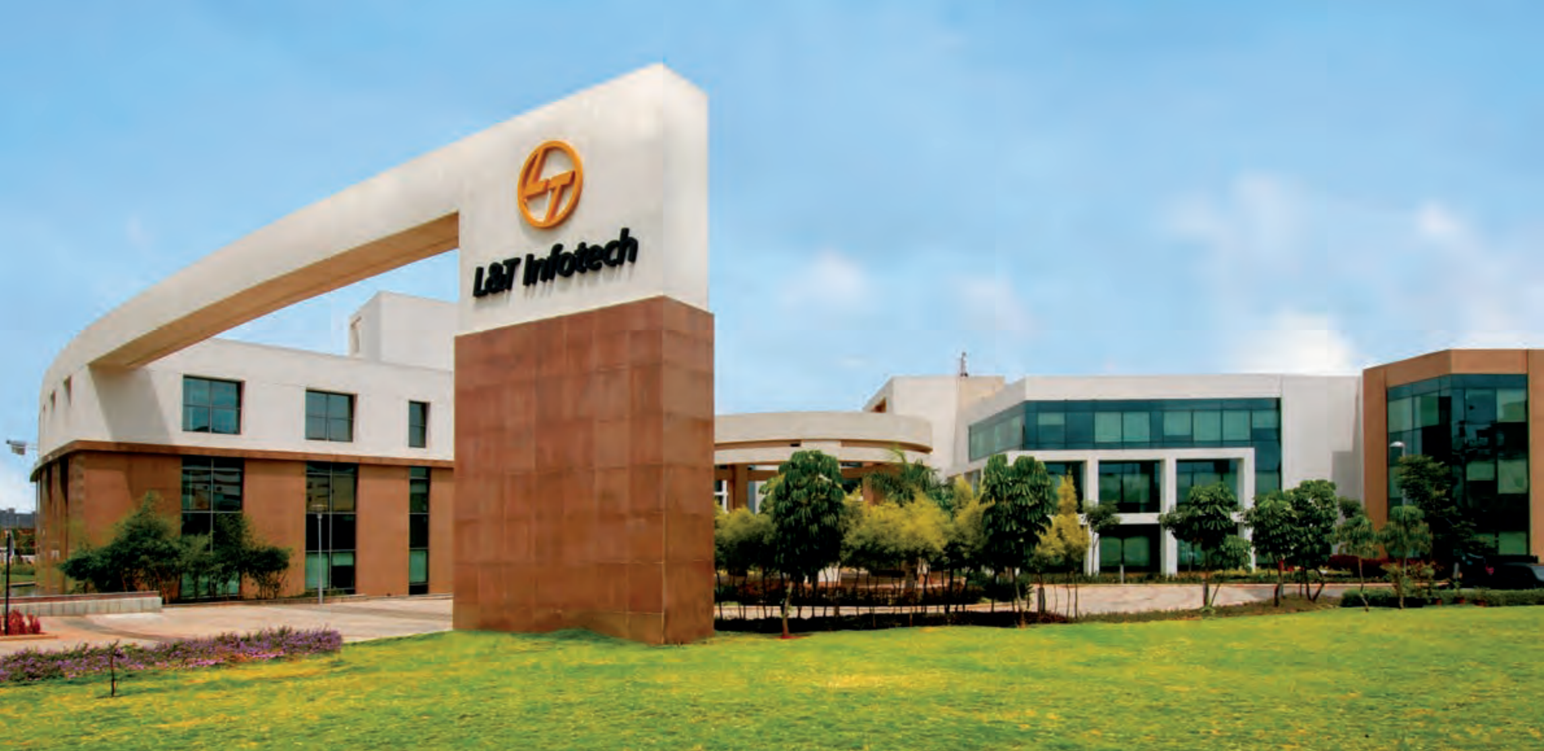
The Bangalore facility of L&T Infotech. This L&T subsidiary offers domain-led solutions to global clients in BFSI, manufacturing, energy and the petrochemical industry.
