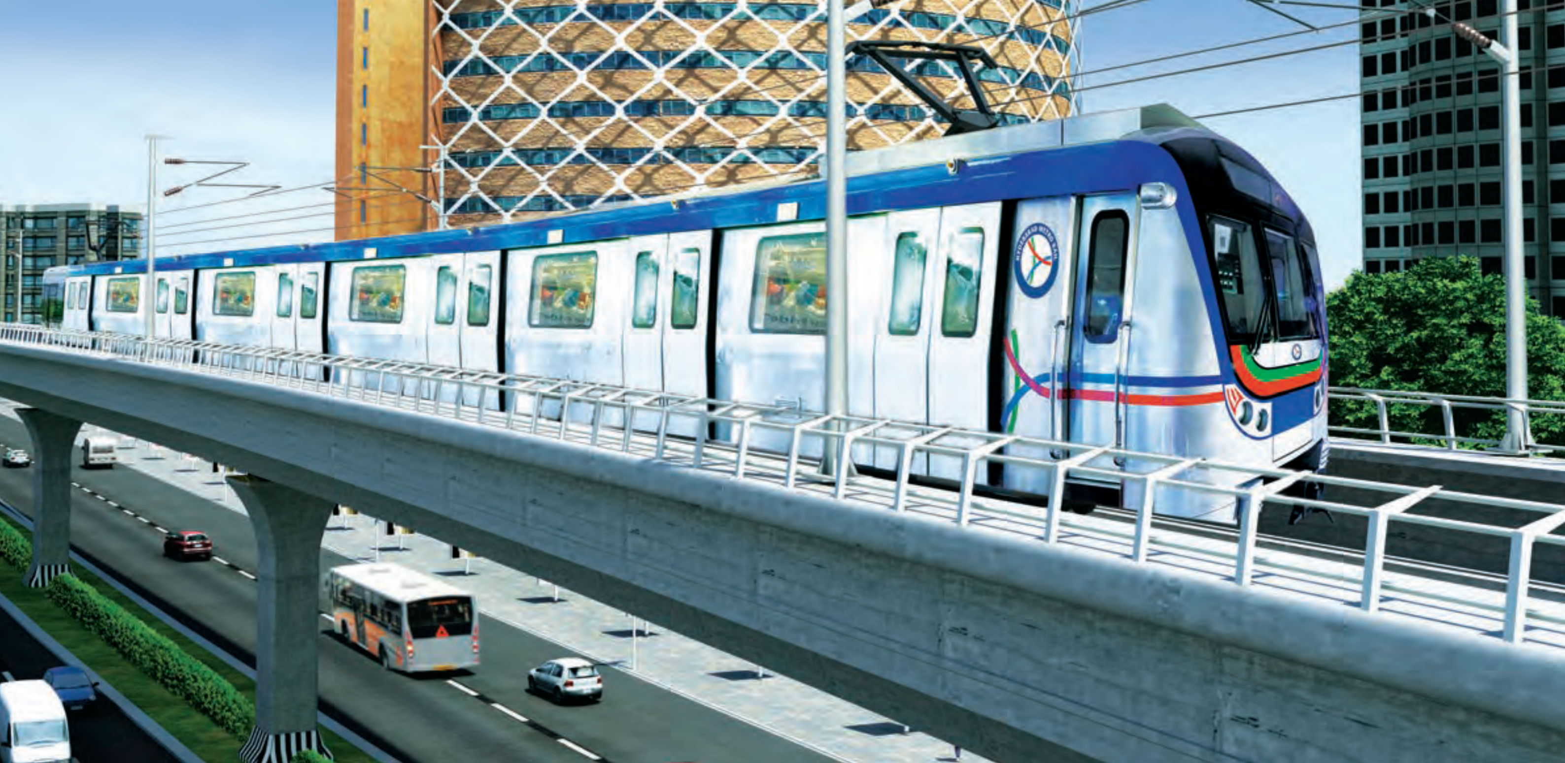
The Hyderabad Metro Rail Project is the world's largest public-private project in the urban transportation sector. It is poised to reduce commuting time and enhance the quality of life in the metropolis of Hyderabad.
