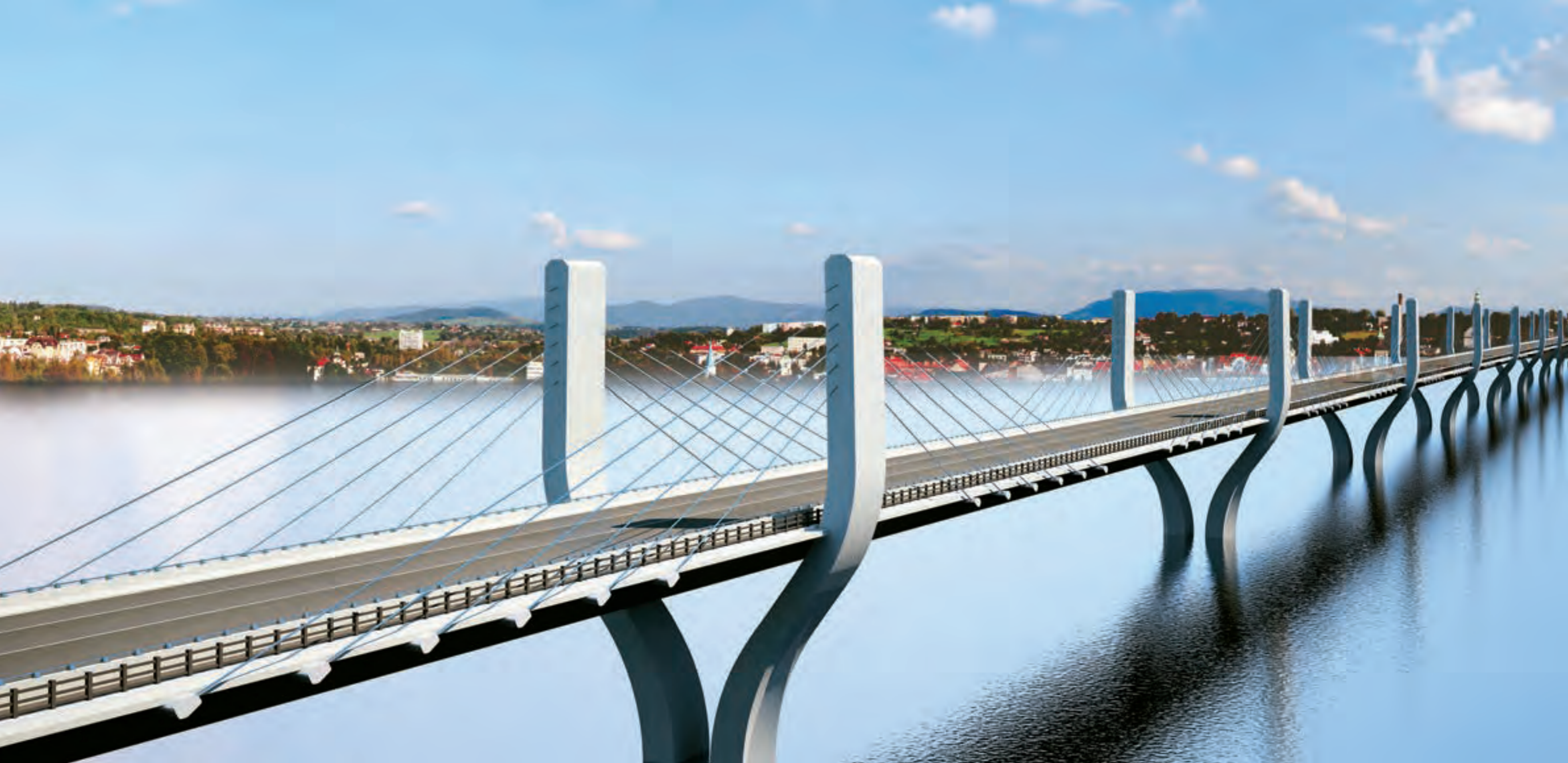
Perspective view of India's longest (1.344 km) extra-dosed, cable-stay bridge across river Narmada in Gujarat. L&T's capabilities include design and construction of many types of bridges of different spans using innovative techniques and construction methods.
