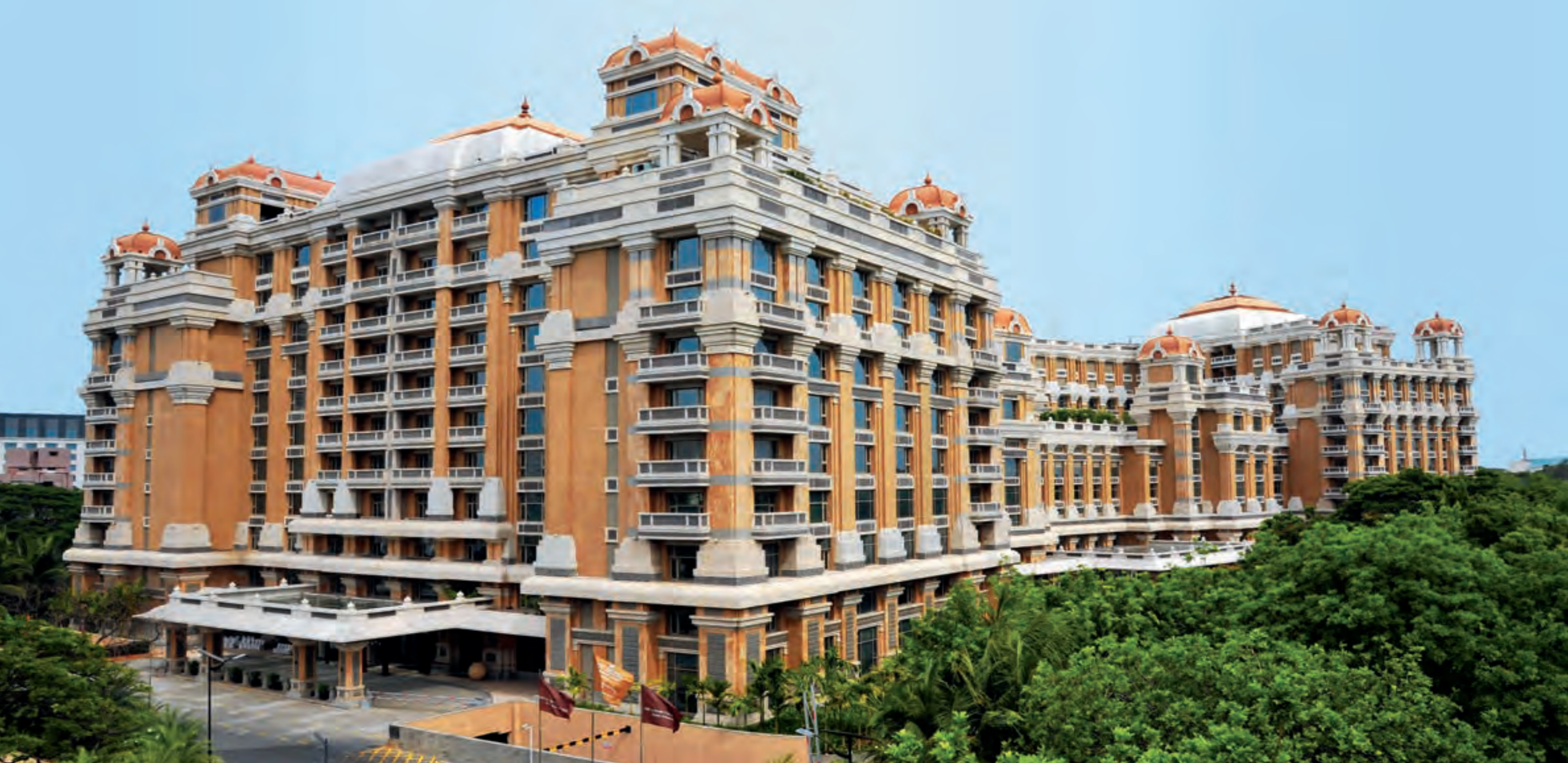
Hotel 'ITC Grand Chola' at Chennai - one of many large luxury hotels built by L&T utilising its end-to-end construction capabilities.
