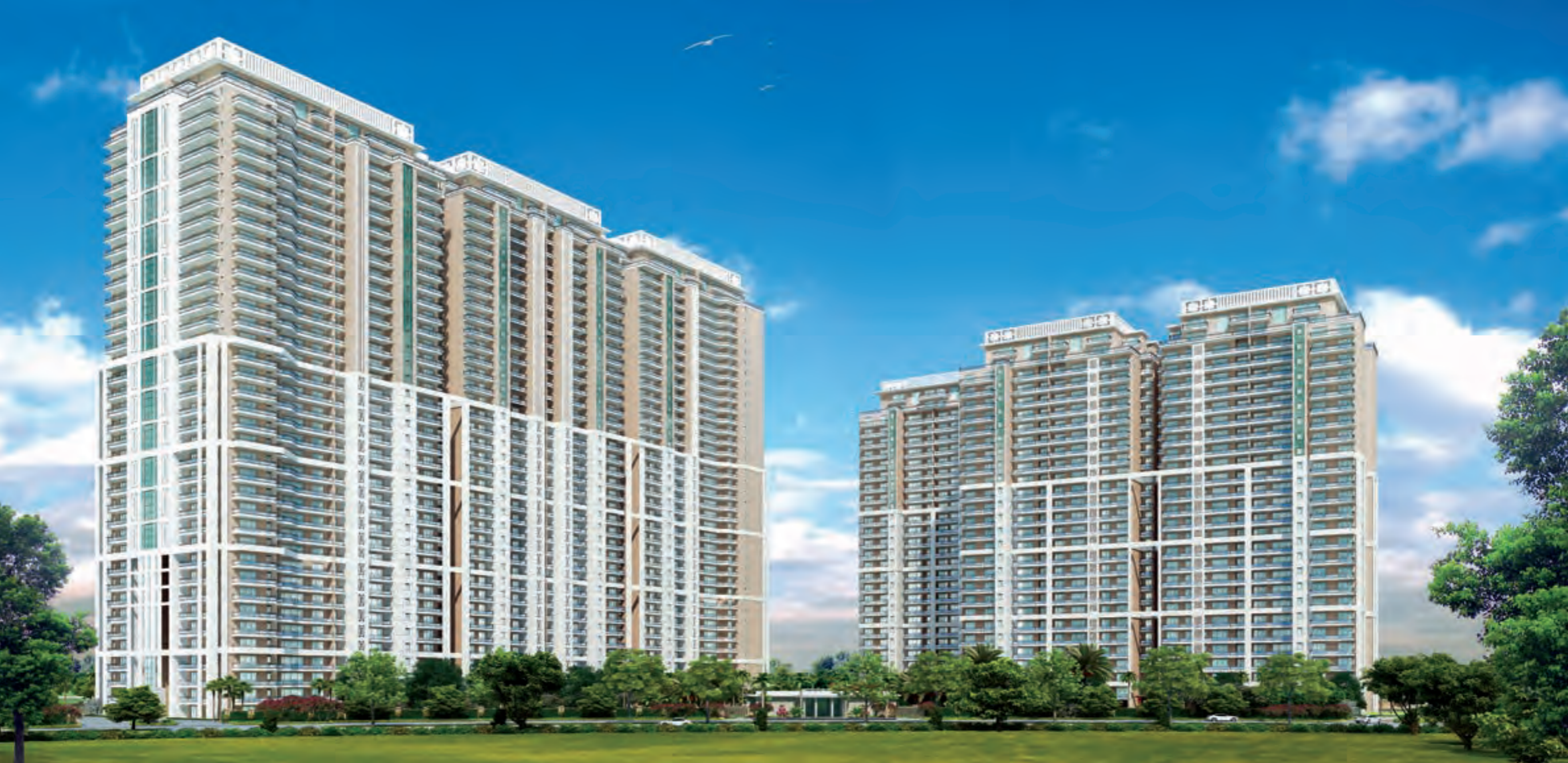
High-rise towers for a residential project in Delhi. The Buildings & Factories business provides world-class 'Concept to Commissioning' solutions across various business segments.
