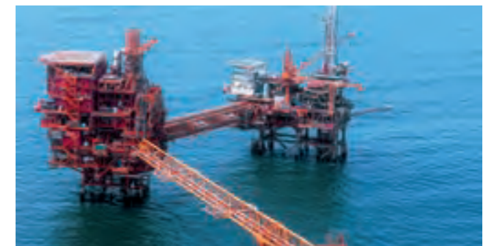
DDW1 Wellhead Platform & Process-cum-living quarters platform for GSPC installed off India's east coast.
