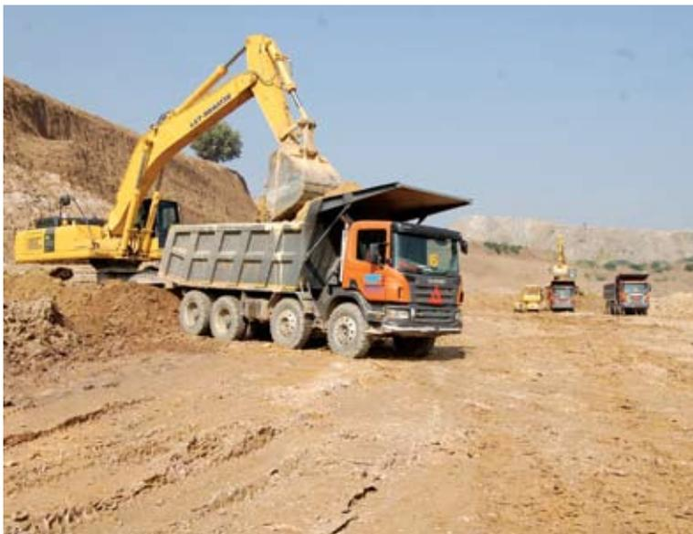
Scania P380 Tipper Truck being loaded by L&T-Komatsu PC450LC-7 Hydraulic Excavator at Sadbhav Engineering site.
