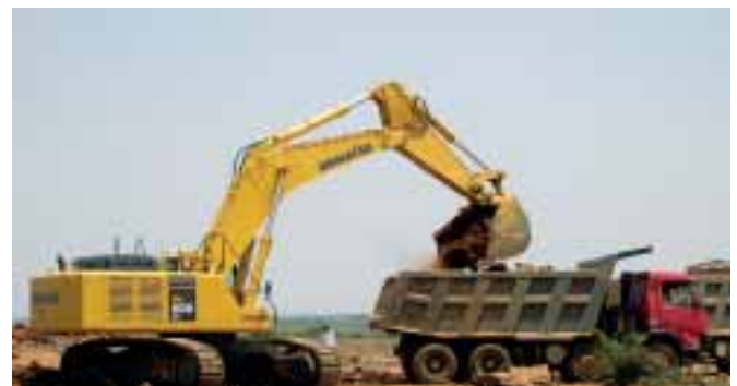
Komatsu PC600 LC working at the Canal Site
