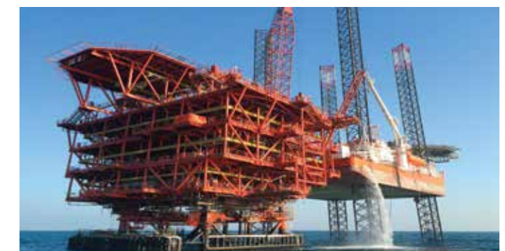
Wellhead platform commissioned off Abu Dhabi.
