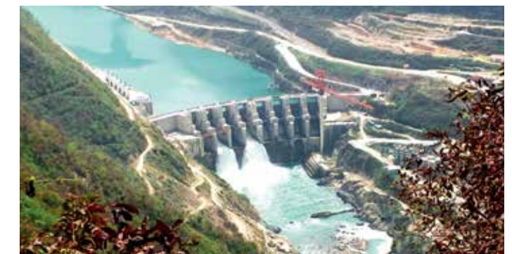
Hydroelectric power plant at the foothills of the Himalayas.
