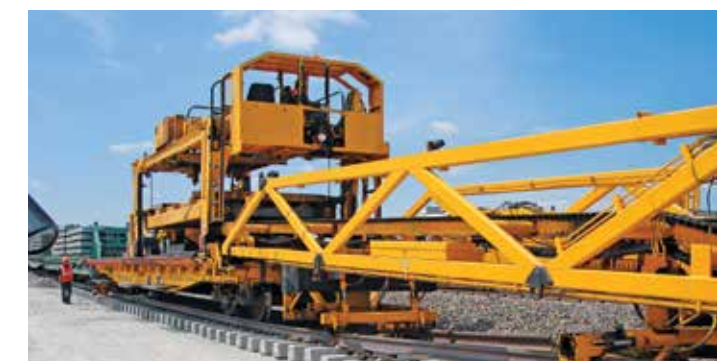
Automated track-laying machine deployed at the prestigious Dedicated Freight Corridor project.
