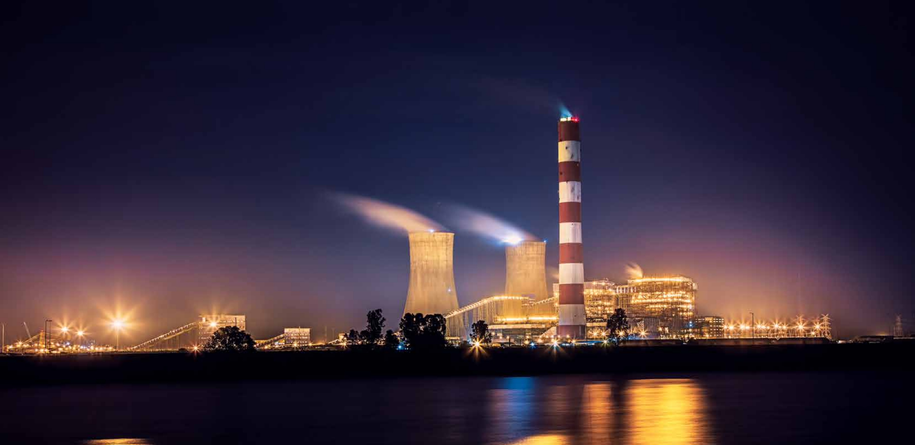
2x700 MW supercritical thermal power plant, Rajpura, Punjab. L&T leverages global technology to provide EPC solutions for thermal power projects across India.
