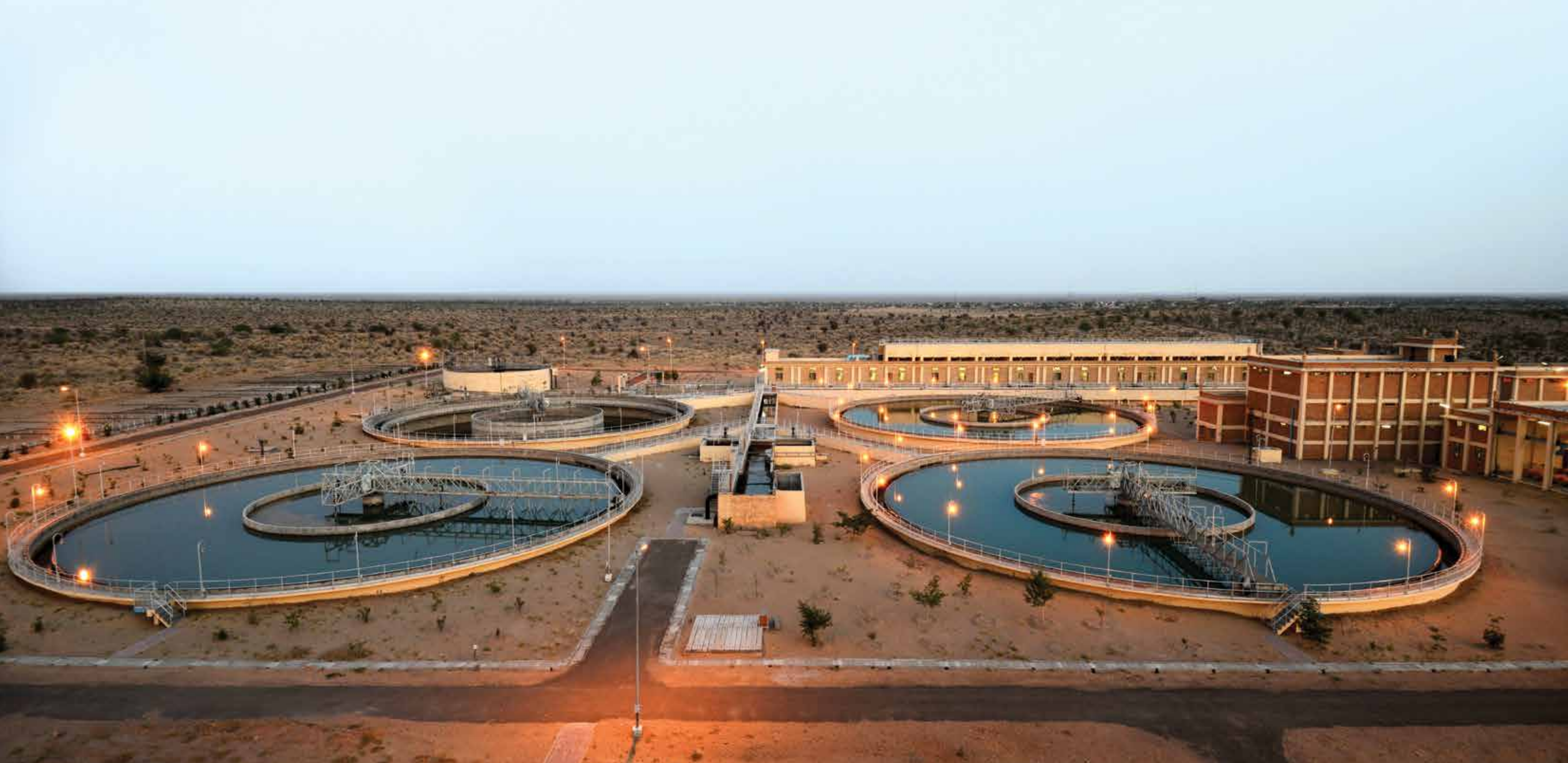
172 MLD Lift Water Supply Project, Jaisalmer, Rajasthan. L&T has designed and constructed water reservoirs, pumping stations, pipeline networks and distribution systems for the water sector.
