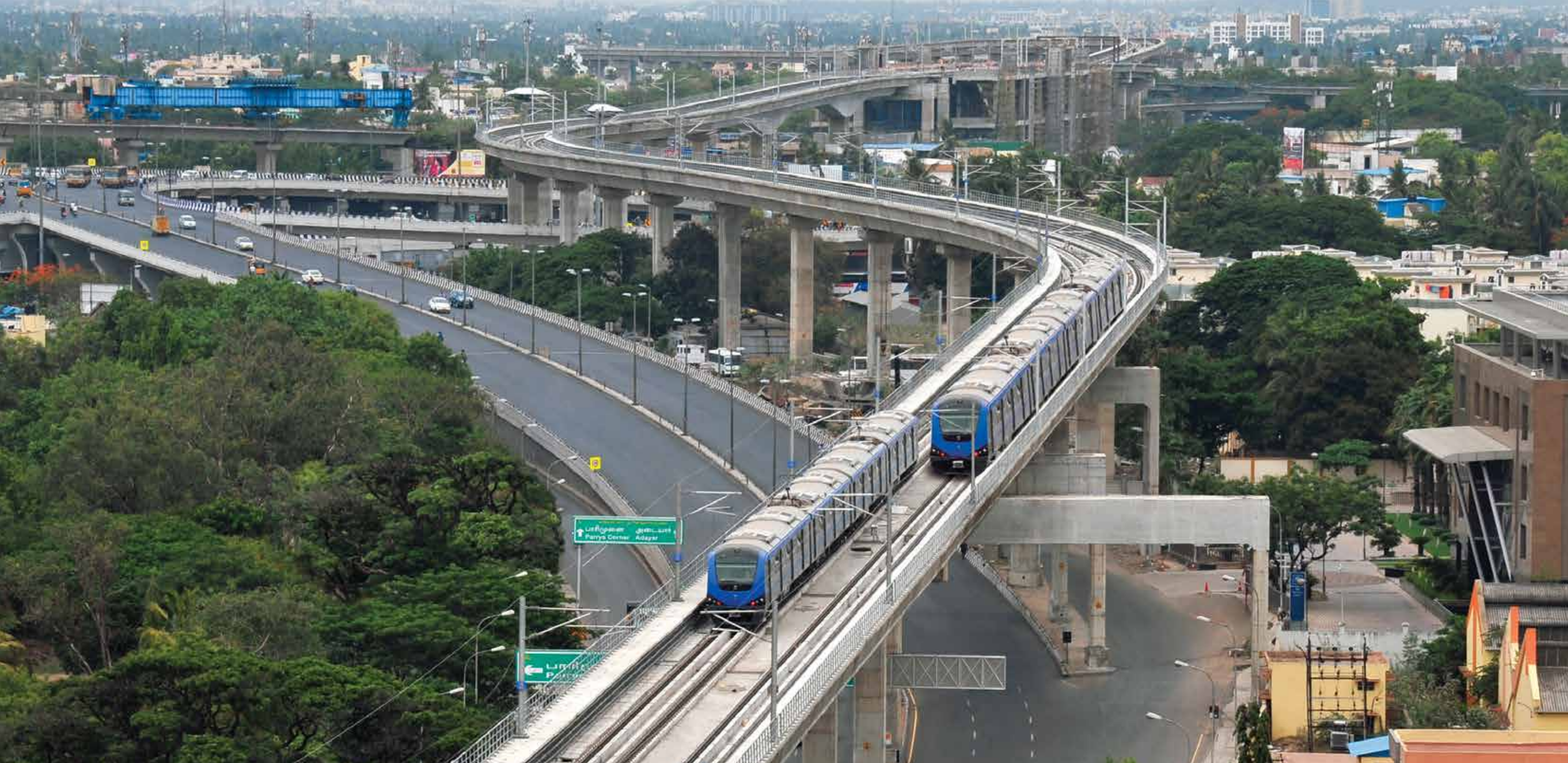
L&T's construction expertise has been offered for the elevated and underground sections of Chennai Metro including ballastless track work and a massive depot. The Company has been engaged in creating robust portals of connectivity for mass rapid transit systems in most of India's major cities - Delhi, Mumbai, Kolkata, Hyderabad, Bengaluru - and soon in Kochi and Lucknow.
