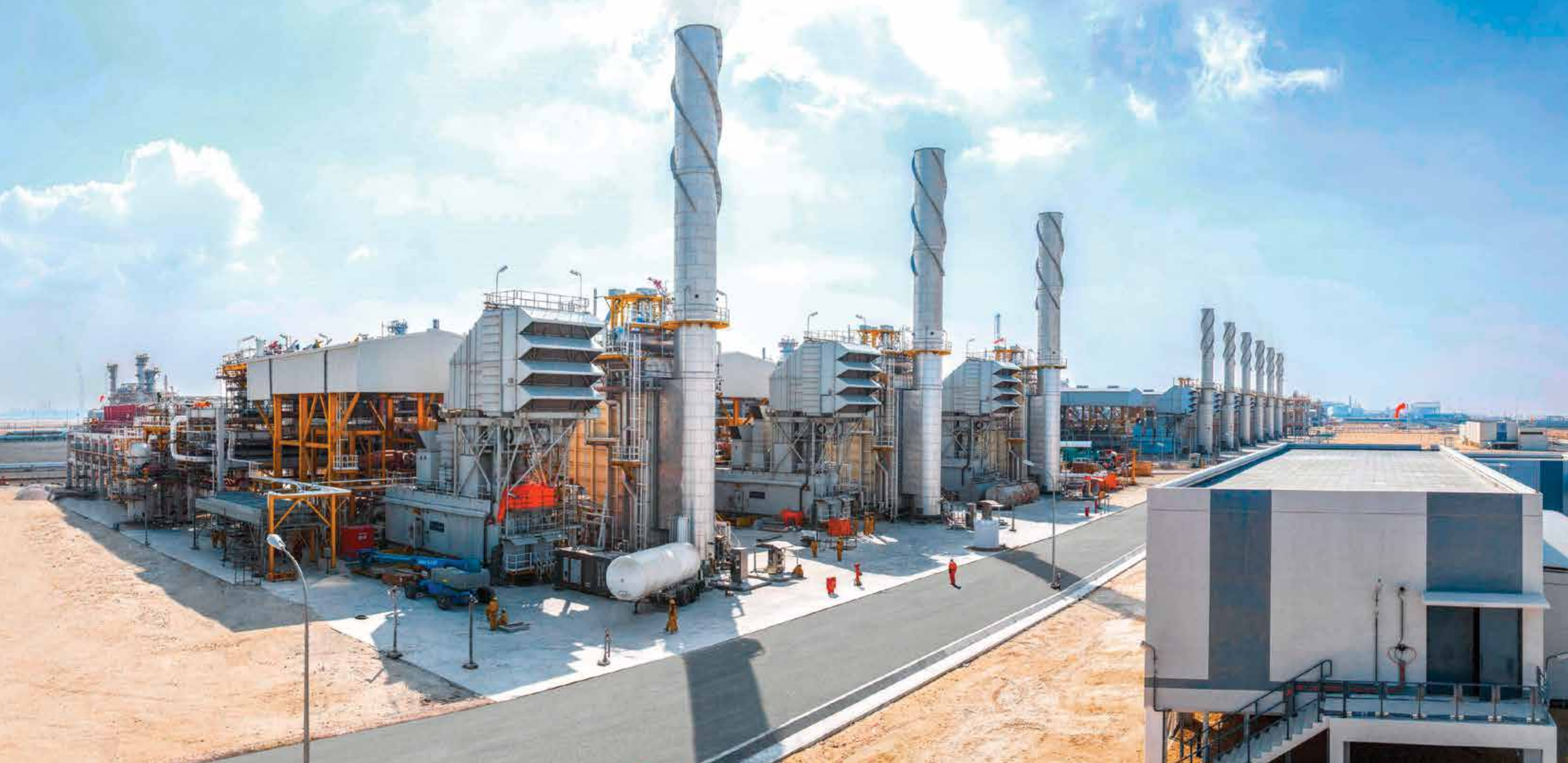
Upgrade project executed on an EPC basis for export gas compression facilities of Dolphin Energy, Qatar. L&T Hydrocarbon has executed multiple complex gas projects, demonstrating the Company's integrated capabilities in this segment.
