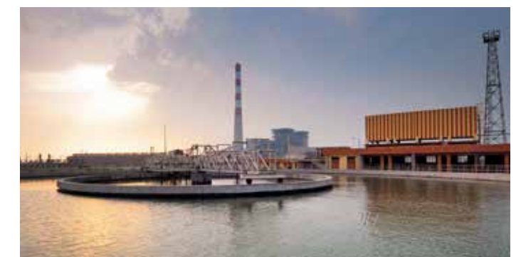
Water pre-treatment plant at Sagardighi, West Bengal.
