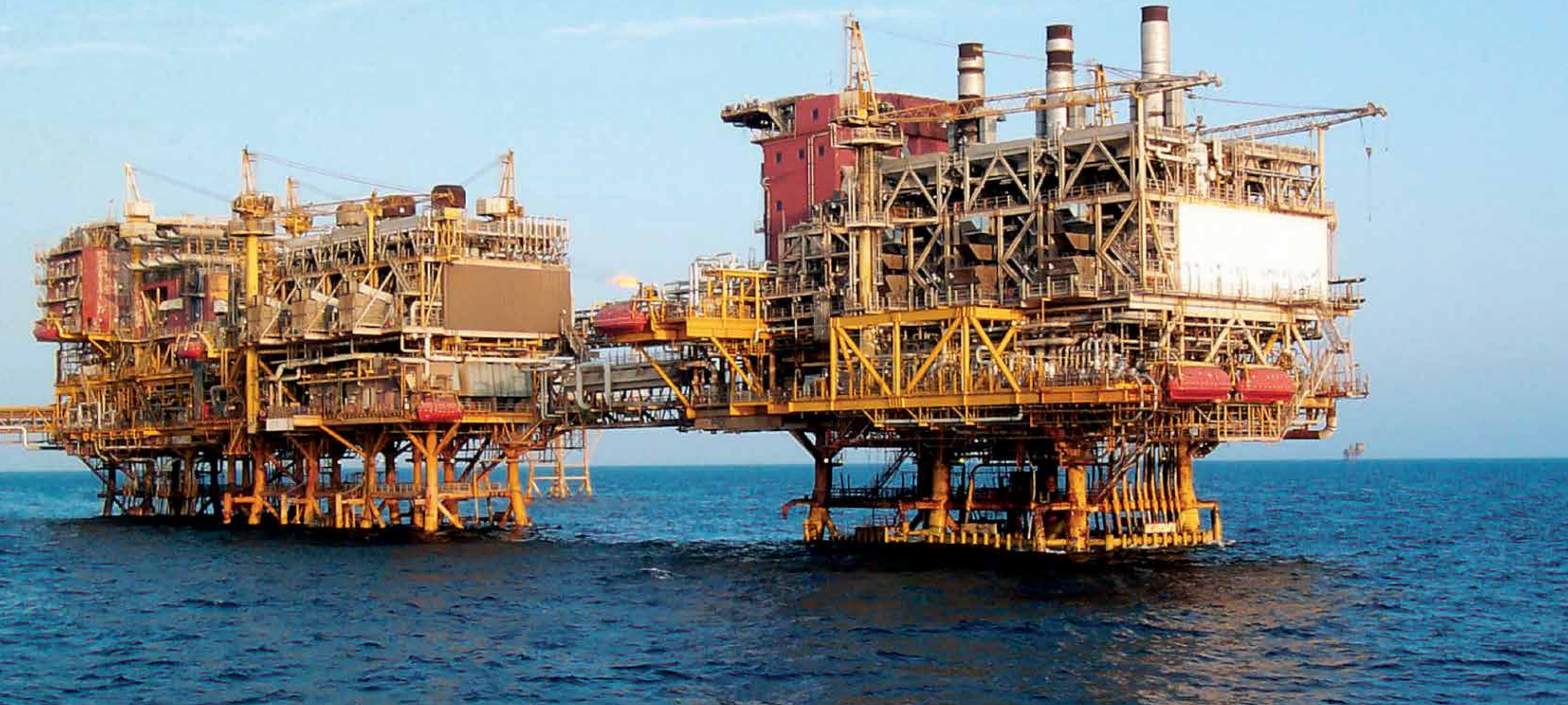
Booster compressor platform with an interconnecting bridge executed for Oil & Natural Gas Corporation (ONGC) in South Basin Gas Fields off India's west coast. This project won the 'PMI Distinguished Project Award' from Project Management Institute, USA.
