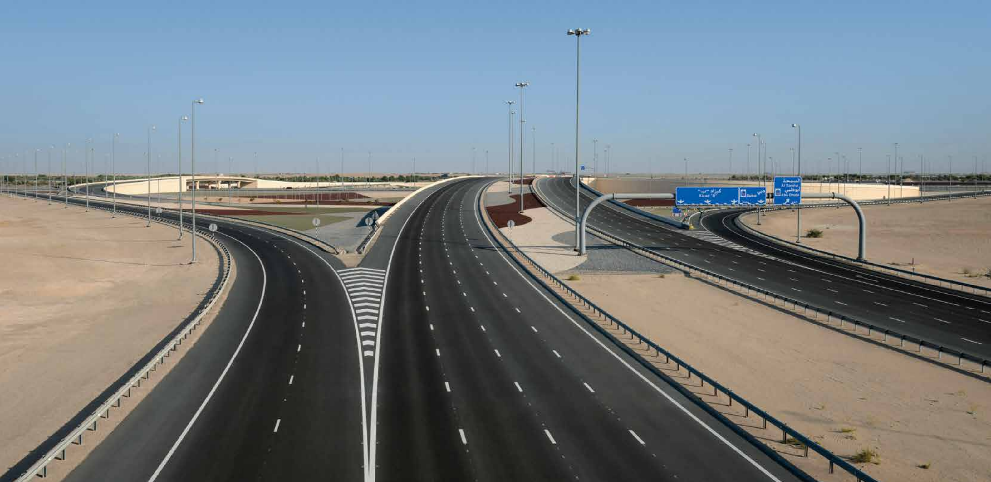
The Sheikh Khalifa Interchange linking the Emirates of Abu Dhabi and Dubai. One of the many infrastructure projects constructed by L&T in the GCC region.
