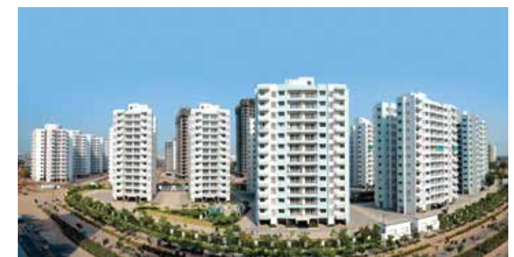
A large residential complex in Ahmedabad. L&T builds residential projects for all segments of society.
