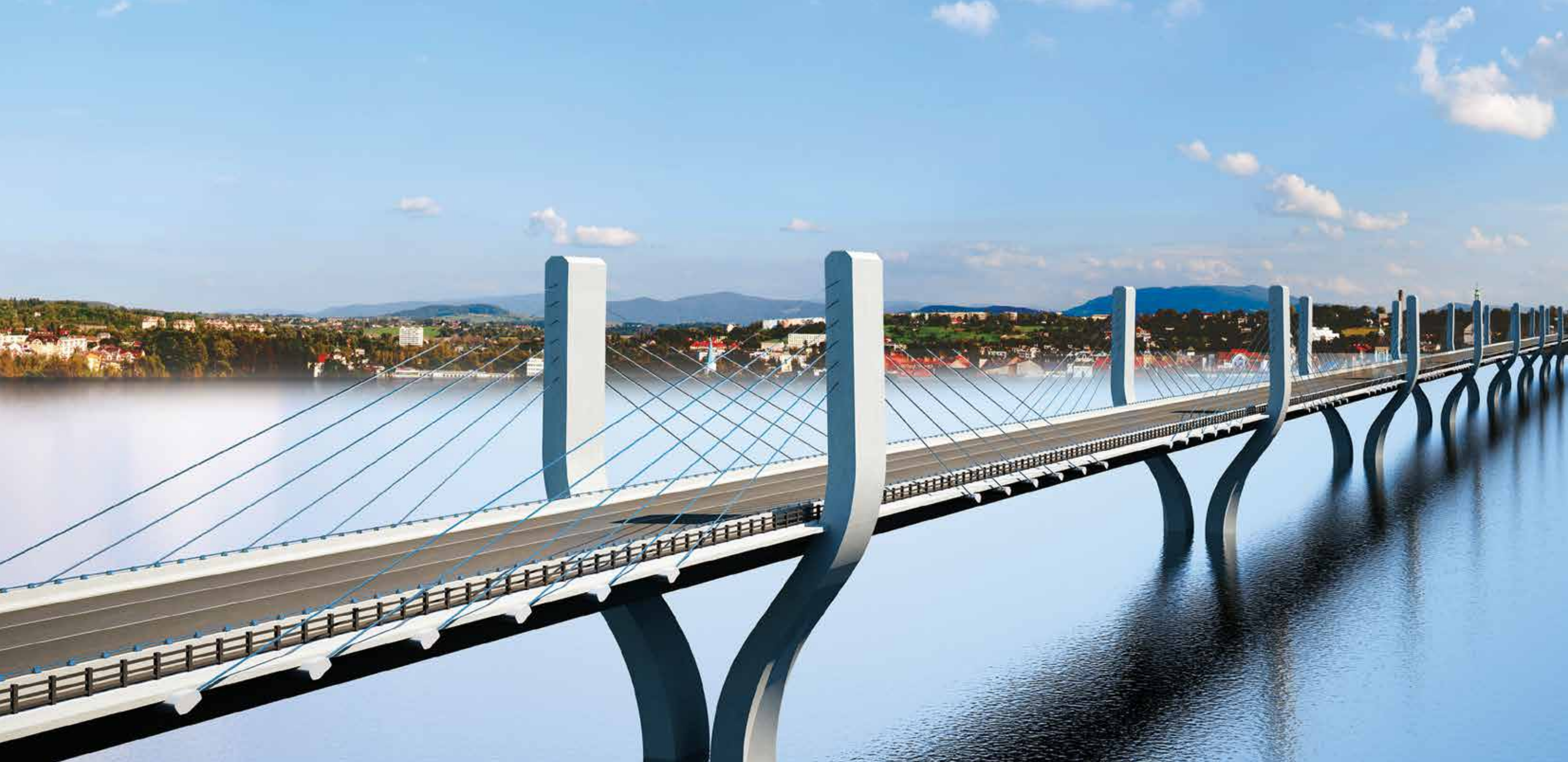
Perspective of the bridge over the Narmada, Gujarat - India's longest extra-dosed, cable stay bridge. L&T's capabilities include design and construction of many types of bridges of different spans using innovative techniques.
