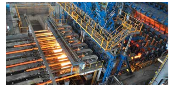
Steel Melt Shop for a steel major in Oman.
