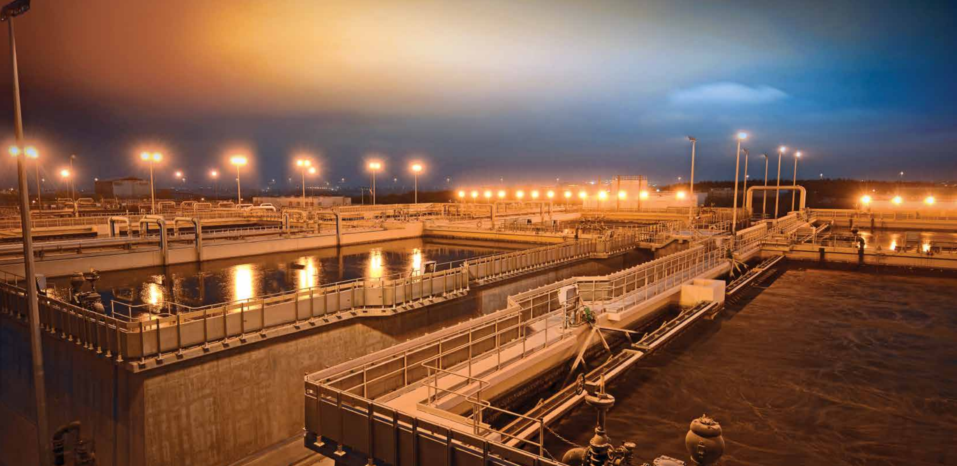
180 MLD waste water treatment plant at Doha, Qatar, deploying SBR technology to boost water sustainability - one of multiple projects that affirm L&T's broad spectrum capabilities in the water sector.
