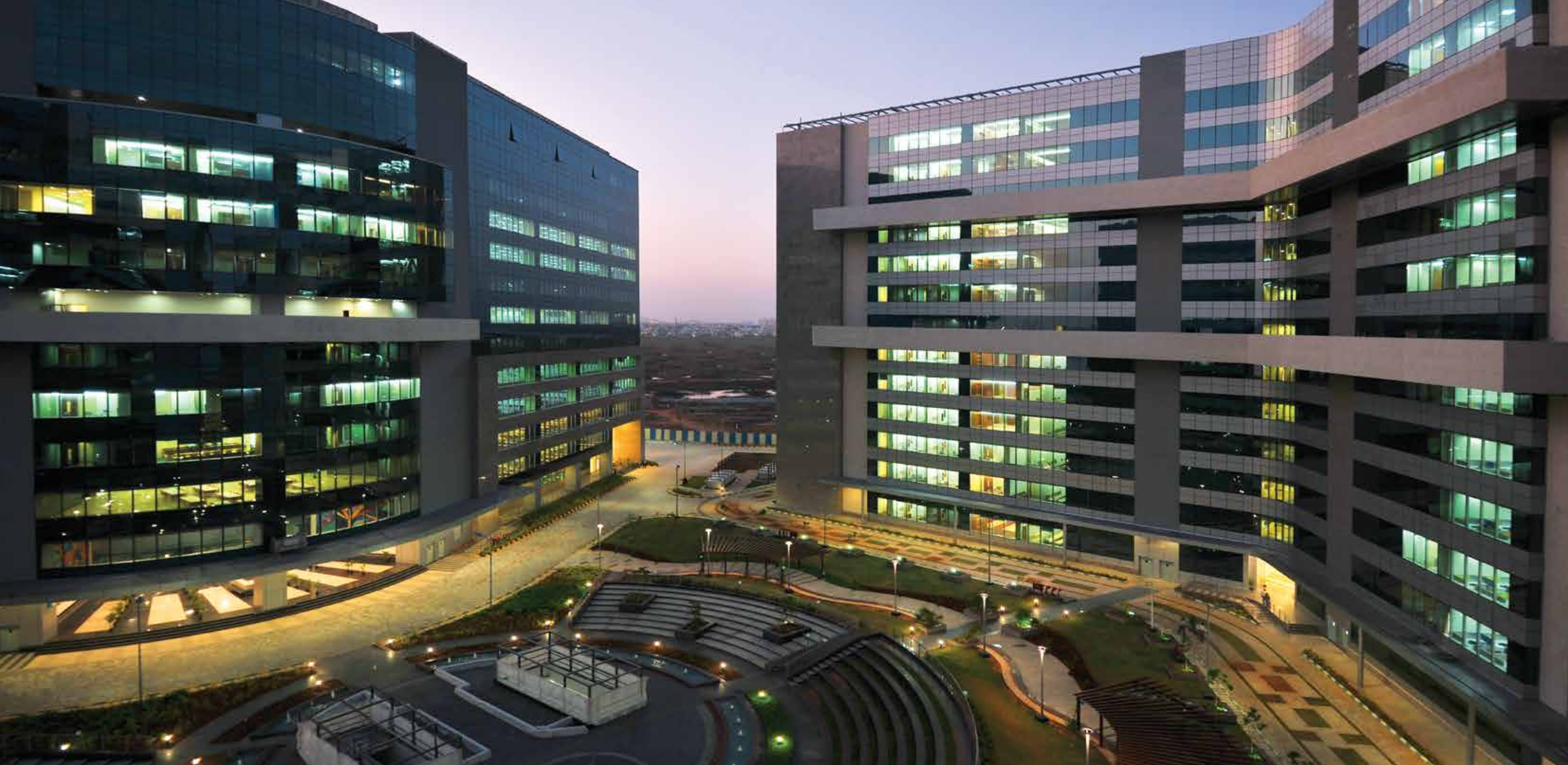
L&T has built over 150 IT parks and commercial complexes in India and neighbouring countries. Total design and construction services enable software companies to just 'plug & play'.
