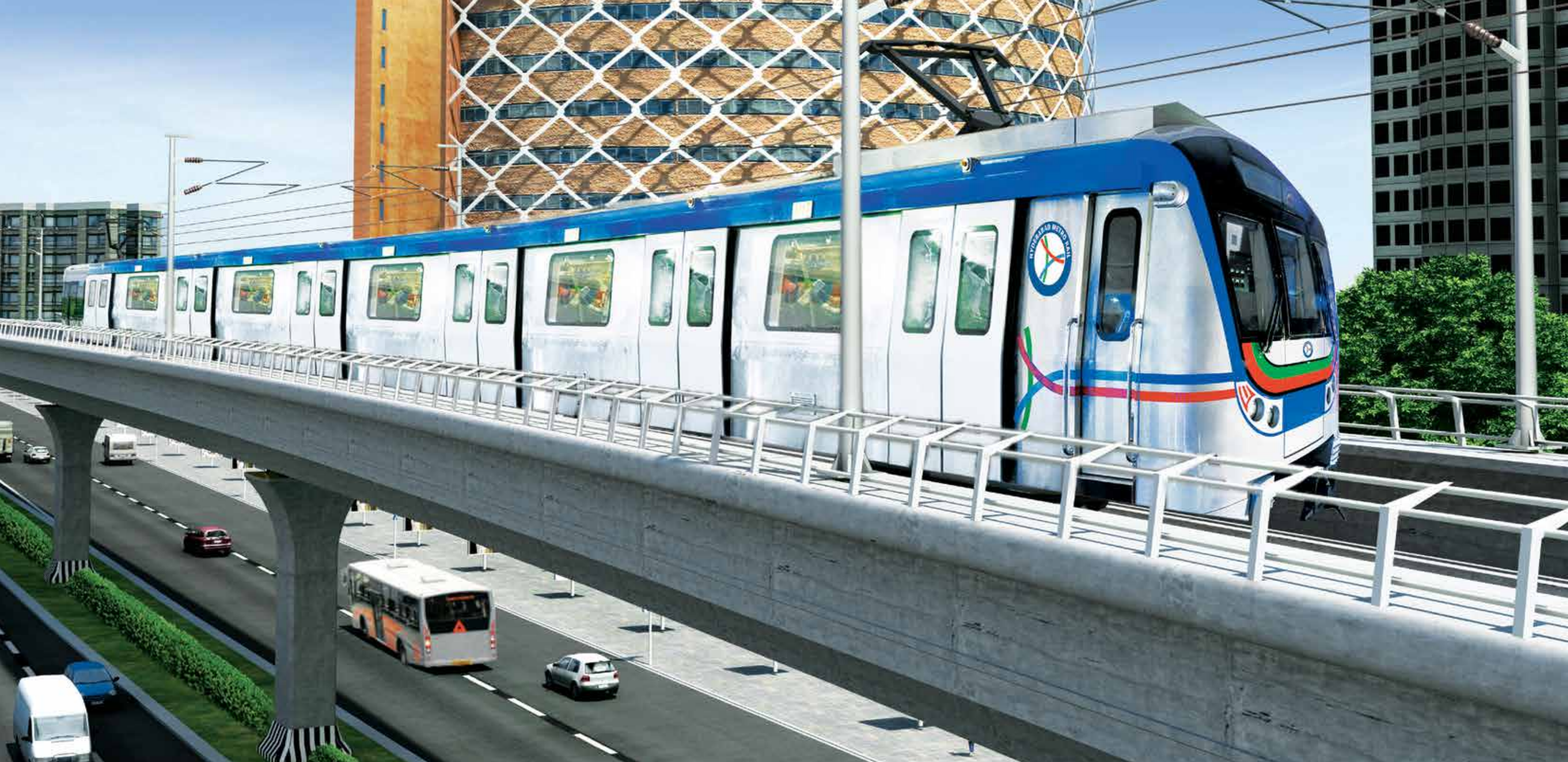
The Hyderabad Metro Rail Project is the world's largest public-private project in the urban transportation sector. Extending 72 km across three corridors, this project is poised to transform life in the metropolis.
