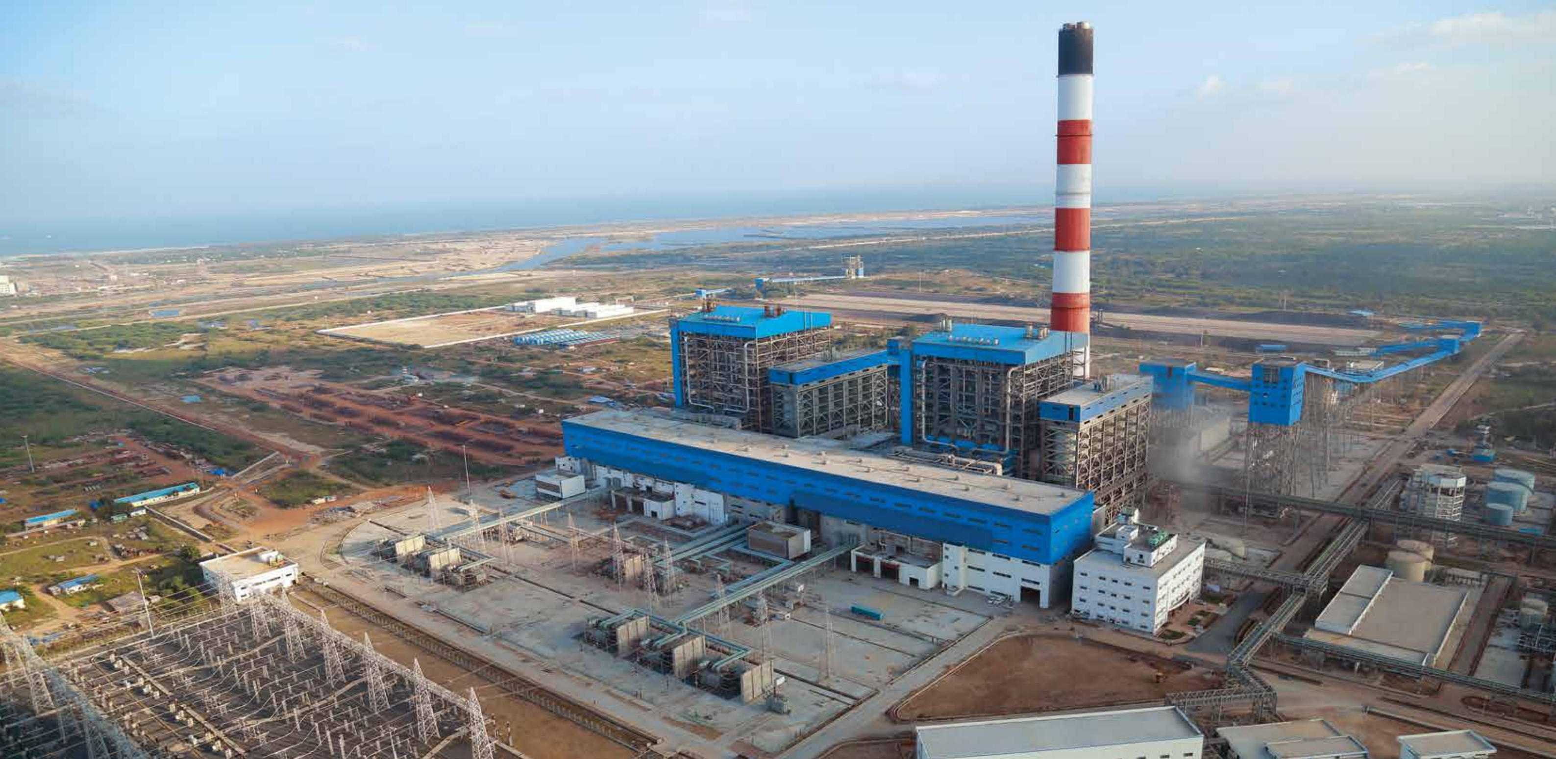
2x800 MW supercritical thermal power plant, Krishnapatnam, Andhra Pradesh. L&T has manufactured critical equipment like turbine-generators, boilers, ESPs and axial fans, among other systems, for supercritical power plants across India.
