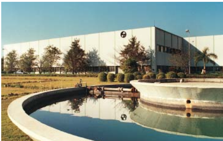
Switchgear Factory, Ahmednagar
