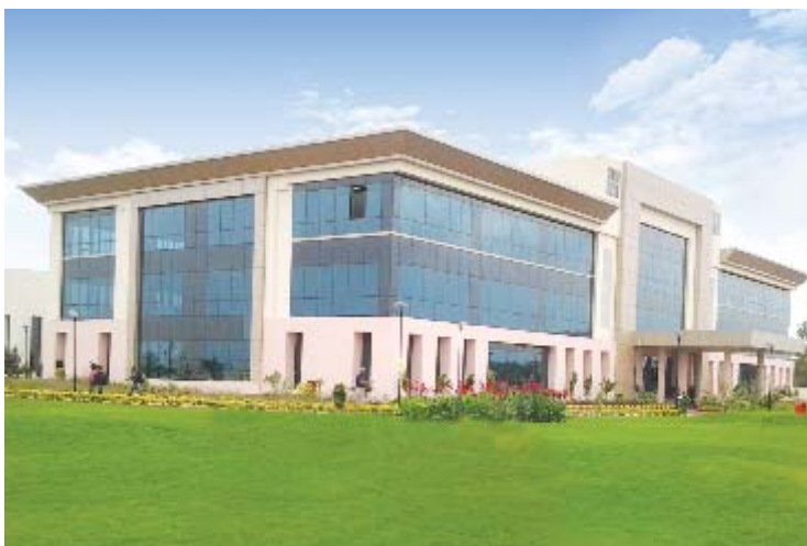
Switchgear Factory, Vadodara
