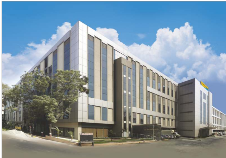
L&T Switchgear Factory - Powai
