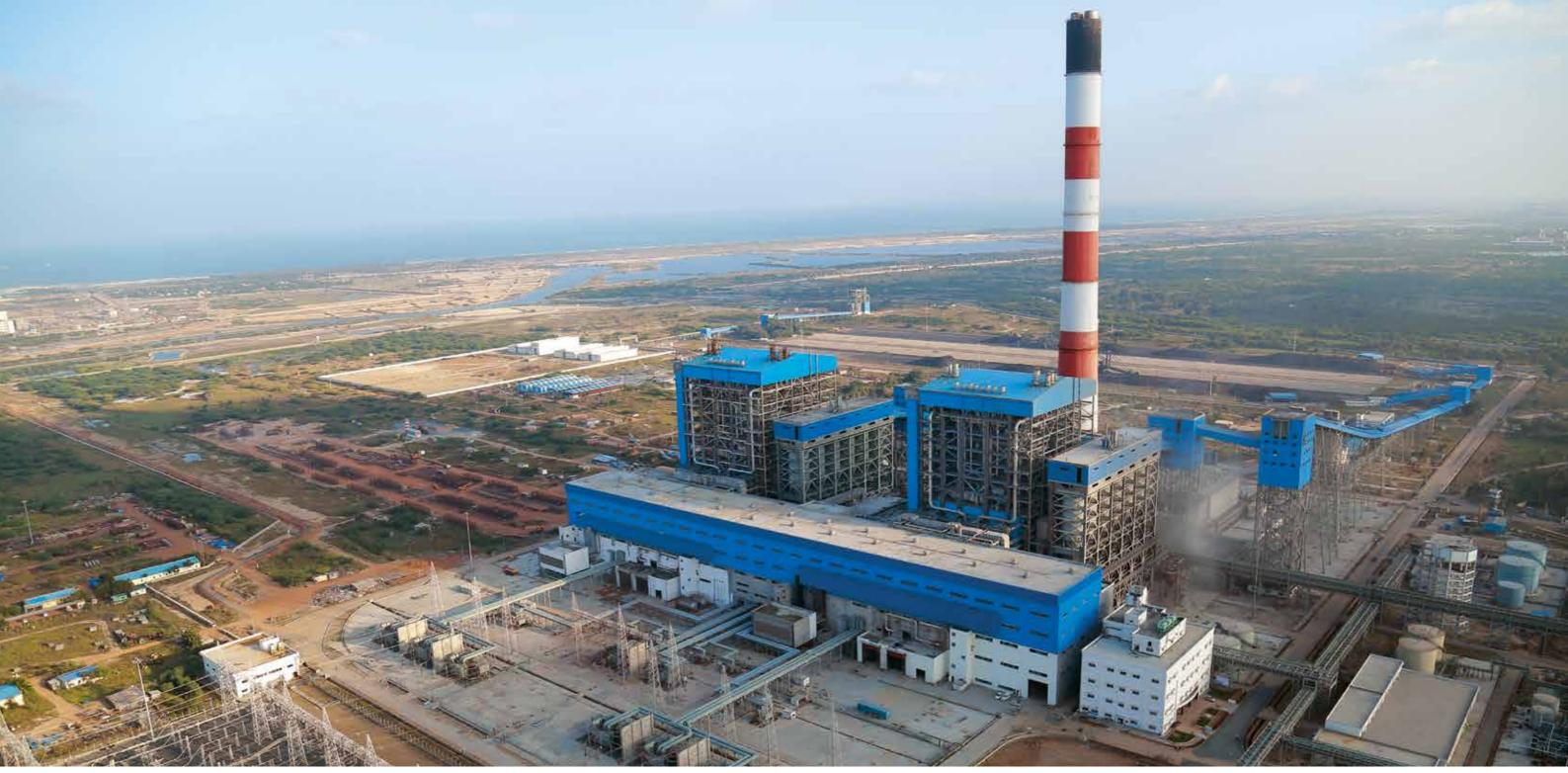
2x800 MW supercritical thermal power plant at Krishnapatnam, Andhra Pradesh. L&T has manufactured critical equipment like turbine-generators, boilers, ESPs and axial fans, among other systems, for supercritical power plants across India.
