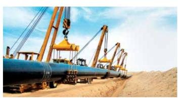
Habshan-Ruwais-Shuweihat gas pipeline project (52" dia x 107 km and 48" dia x 15 km) built on EPC basis for GASCO, Abu Dhabi.
