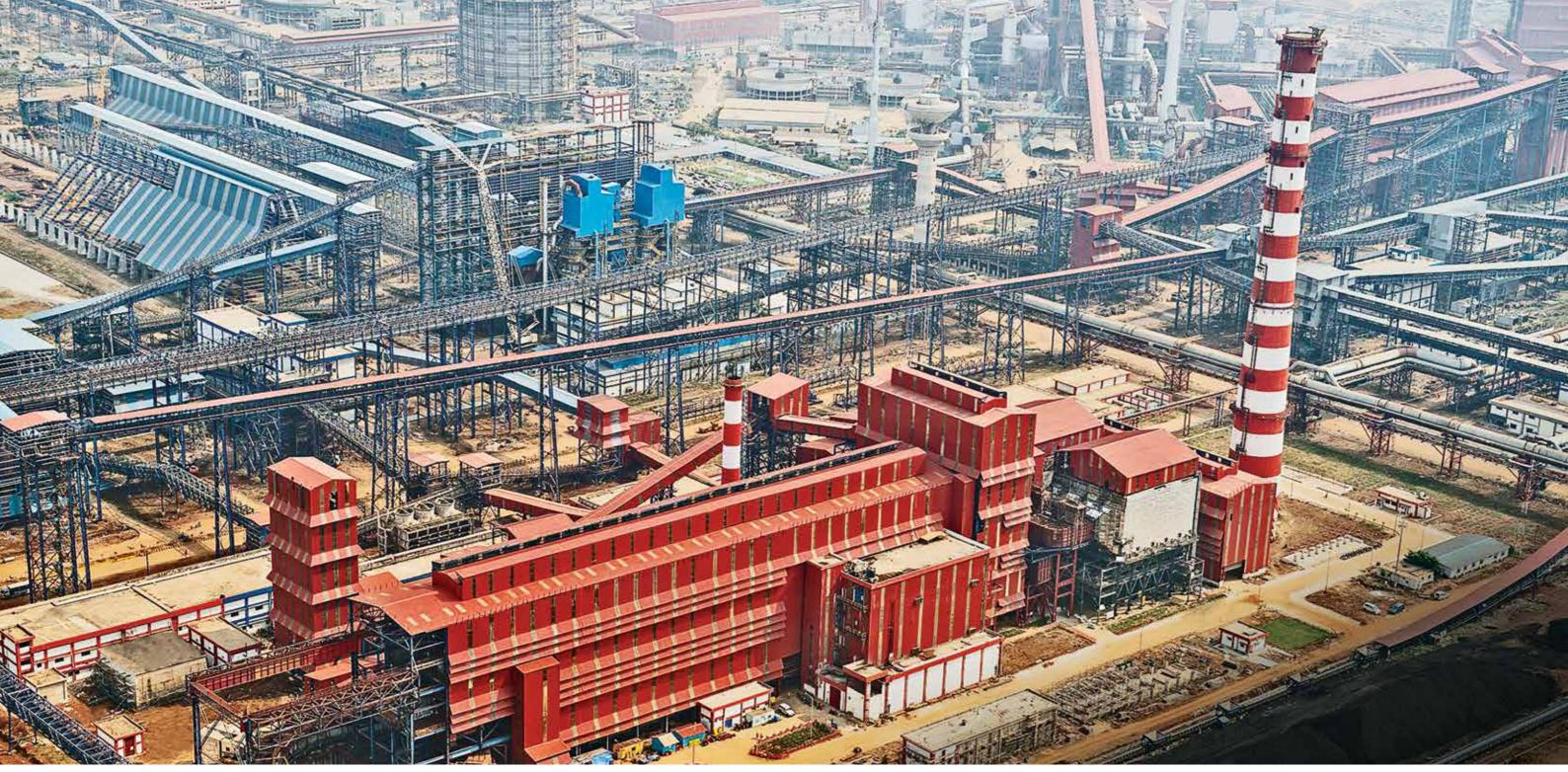
Integrated Steel Plant, Kalinganagar, Odisha. L&T offers steel-makers a single dependable source for services ranging from engineering to commissioning of blast furnaces, sinter plants, pellet plants, coke oven batteries, etc.
