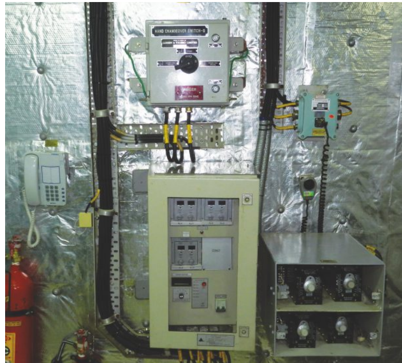
Onboard Installation of electrical components including cabling and lighting
