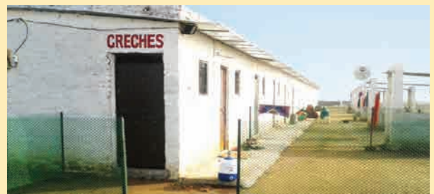
Crèche facility for children of workmen
