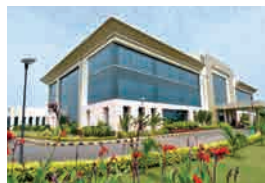
Administrative Building, Vadodara
