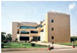
Administrative Building, LTSSHF, Hazira
