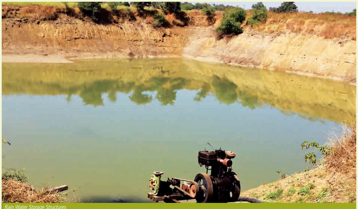
Rain Water Storage Structures
