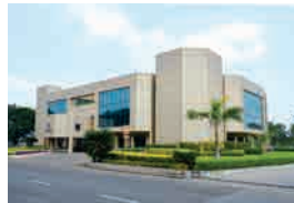
SBU Block (2 nd floor), Hazira
