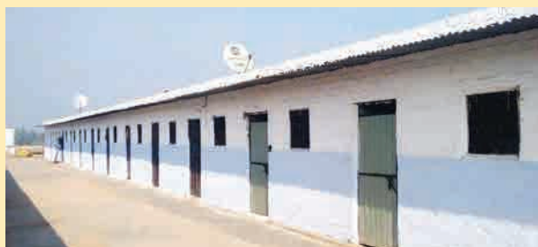
Comfortable accommodation at Workmen's Camp
