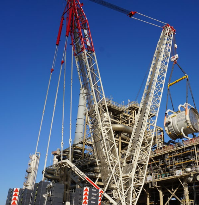
Heat Train Exchanger Replacement at Kuwait
