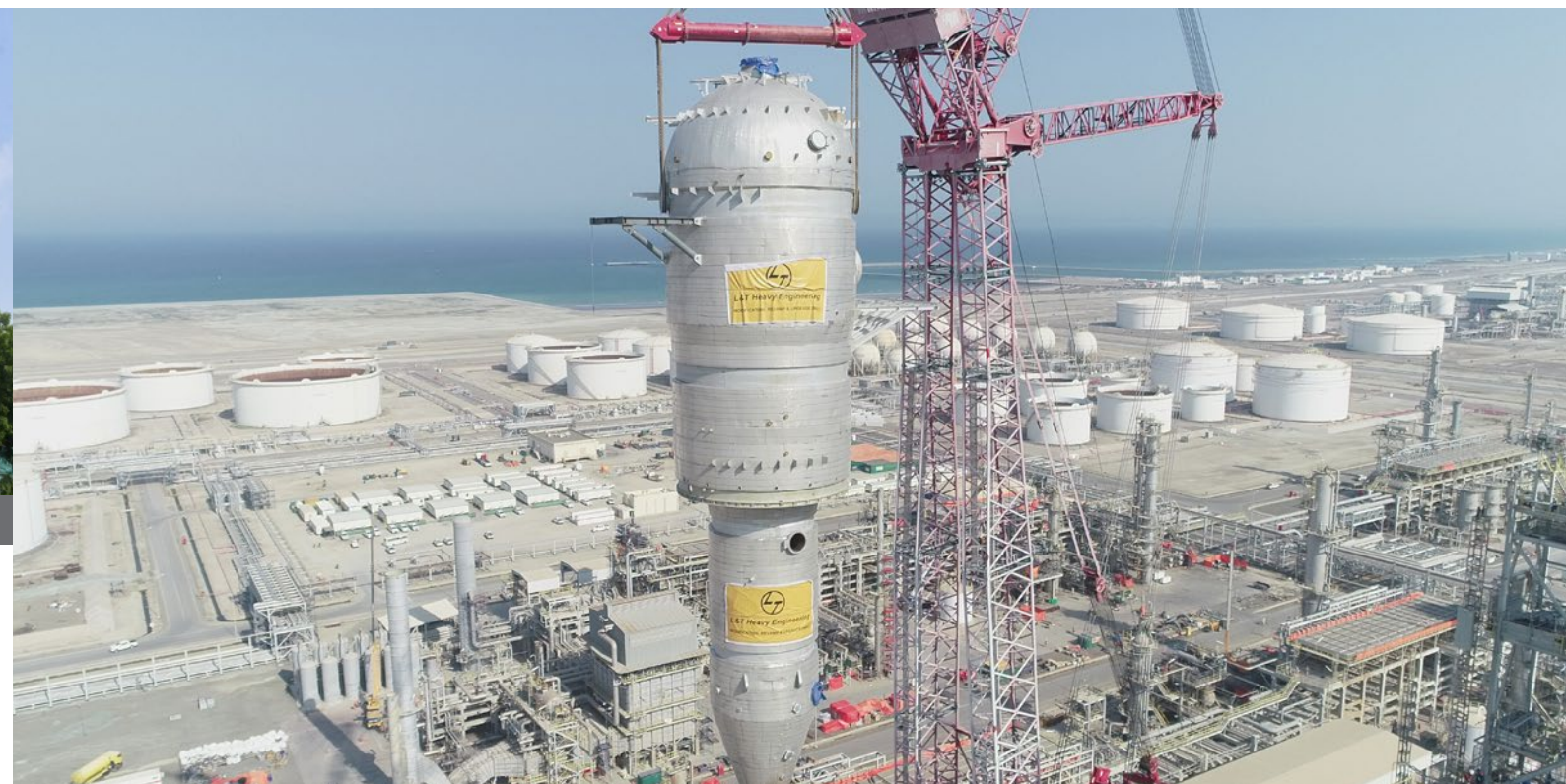
Replacement of FCCU Reactor with Internals for OQ at Oman
