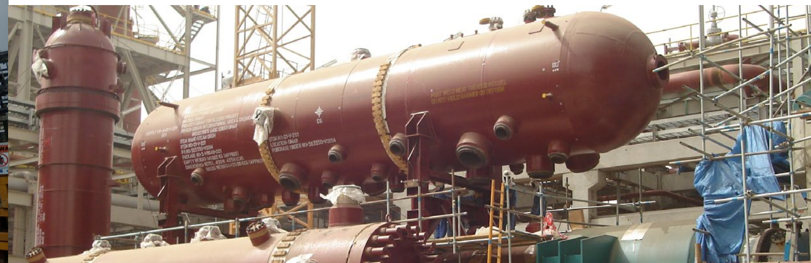
Waste Heat Boiler Package including RG/CG boiler, steam drum, risers & downcomers at Sohar Fertilizer plant
