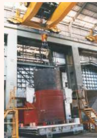
Shrink fitting operation for multi wall construction of Cr-Mo-V reactors
