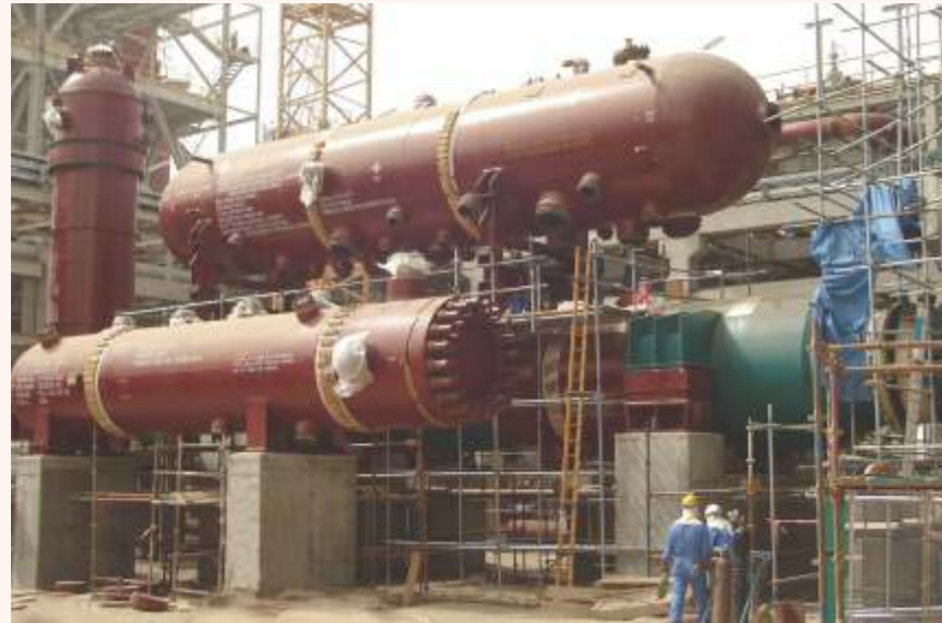
Waste Heat Boiler Package including RG/CG boiler, steam drum, risers & downcomers at Sohar Fertilizer plant
