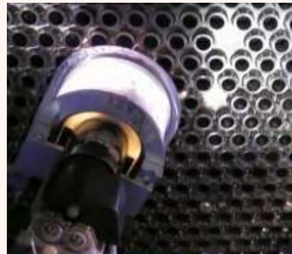
Automatic tube-to-tube sheet welding
