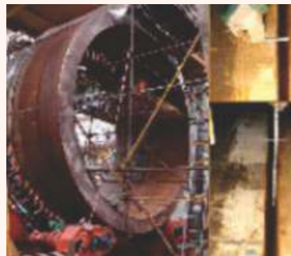
Narrow Gap Tandem SAW on 322mm-thick forged reactor circular seam
