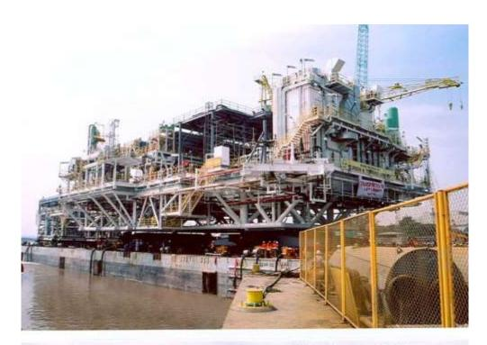
The 2400-tonne process platform built by L&T begins its 2500-km journey from L&T's Modular Fabrication Facility at Hazira, Surat to the El Bunduq oil fields of Abu Dhabi. The giant platform will be installed at site by January 16, 2006 – as part of the \$52.5 million Engineer-Procure-Construct contract secured by L&T.
