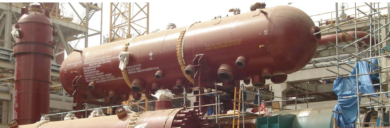
Waste Heat Boiler Package including RG/CG boiler, steam drum, risers & downcomers at Sohar Fertilizer plant
